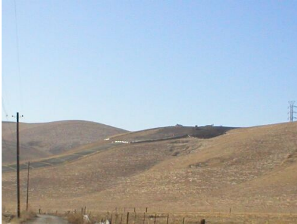
Figure 1 – Transition Station and downslope area, November 22, 2005.
