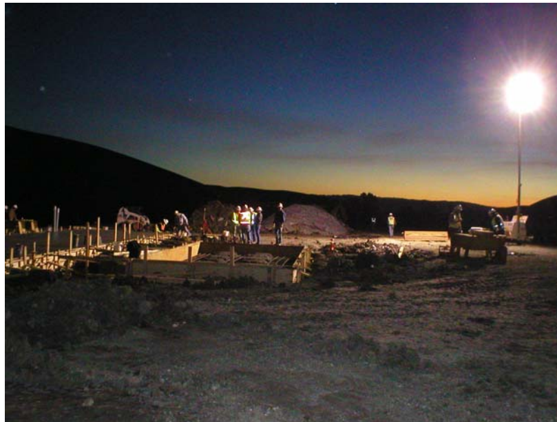
Figure 4 – Night work at the North Dublin Substation, December 7, 2005.
