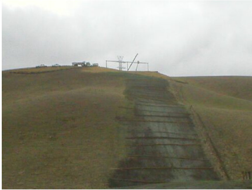
Figure 1 – Crews taking down the top beam from the frame structure at the Transition Station, December 22, 2005.
