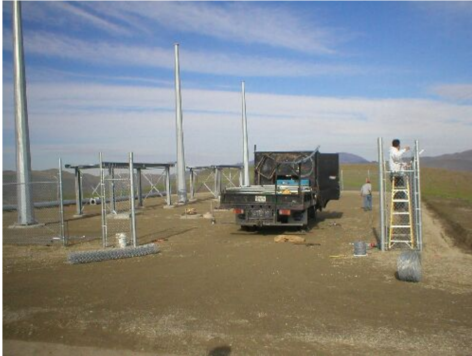
Figure 1 – Fence installation at the Transition Station, January 11, 2006.
