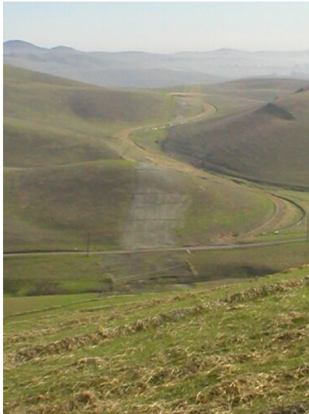
Figure 2 – Road 7 previous landslide area where erosion controls have been fixed, January 11, 2006.
