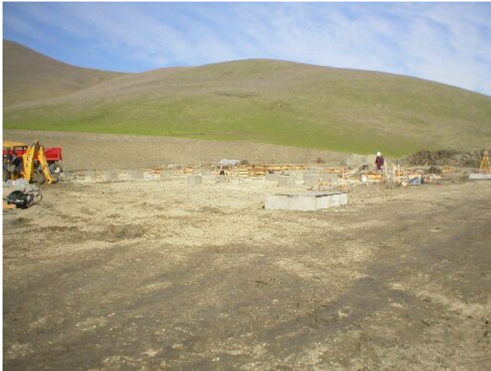
Figure 5 – Foundation structure installation at the North Dublin Substation, January 11, 2006.
