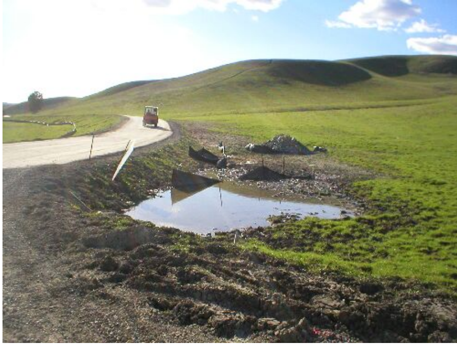
Figure 1 – Poned area adjacent to the Substation ramp prior to draining, February 15, 2006.
