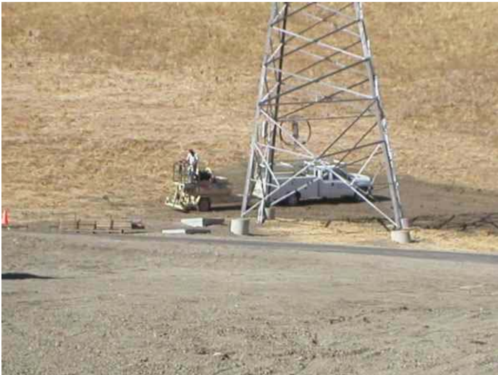
Figure 11 – NVC crews hydro-seeding the graded pad area around Tower #1, October 17, 2006.
