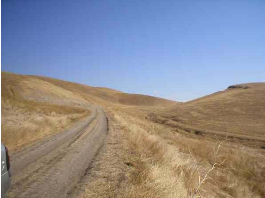
Figure 6 – Cut slope above Vault 7 along Road 7, October 13, 2006.
