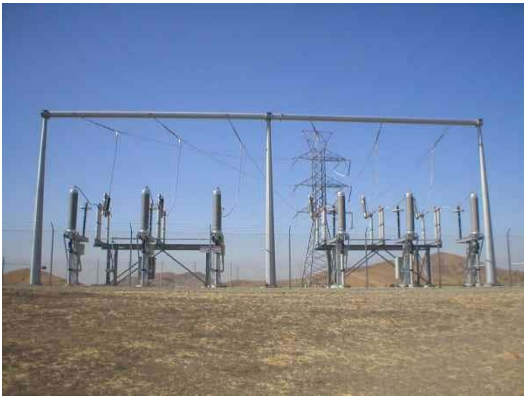
Figure 7 – Transition Station, October 13, 2006.
