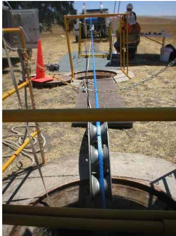
Figure 2 – Line pulling the cable from Vault 3 to Vault 4, June 22, 2006.
