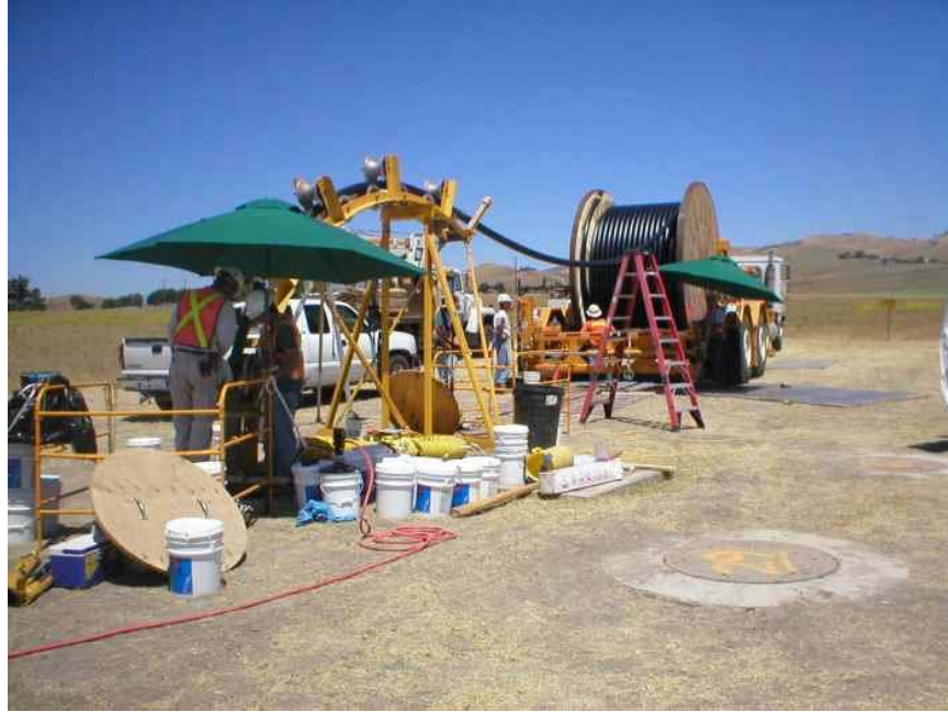
Figure 1 – Cable pulling through installed conduit at Vault 3, June 22, 2006.
