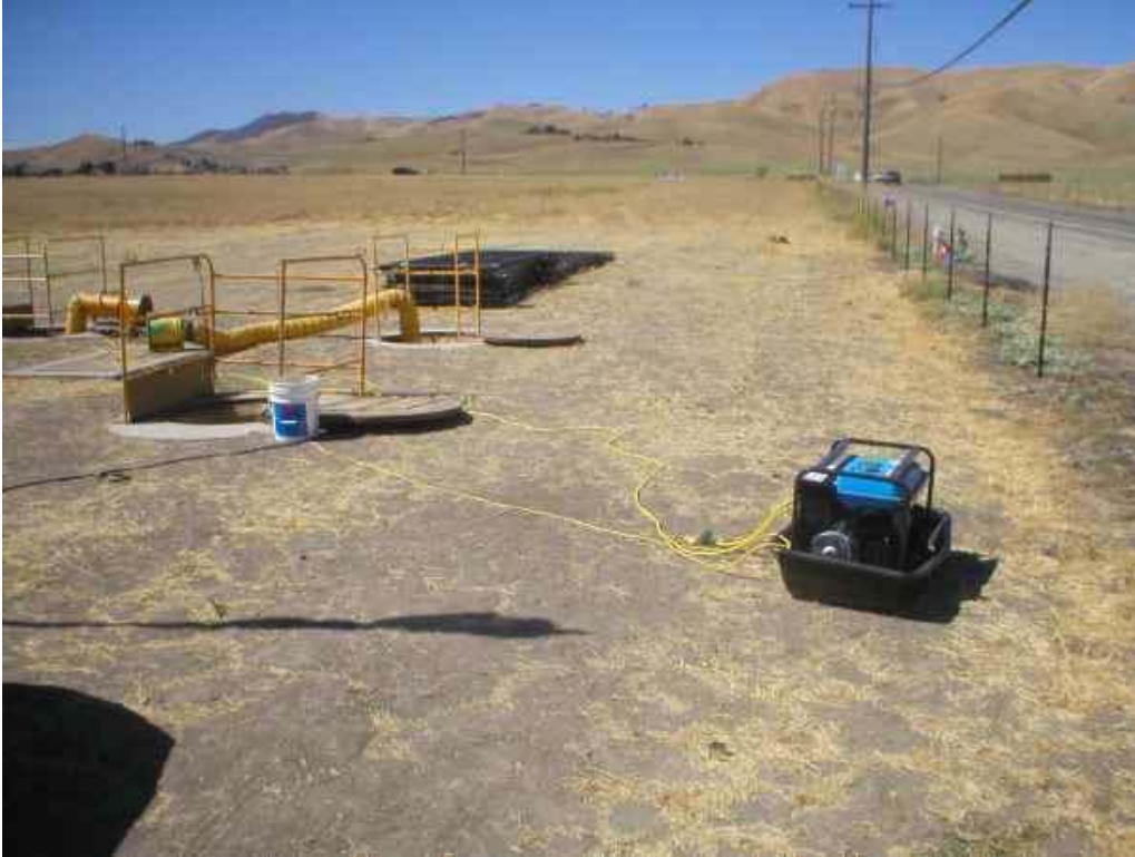
Figure 1 – Cable splicing operations at Vault 3, July 11, 2006.
