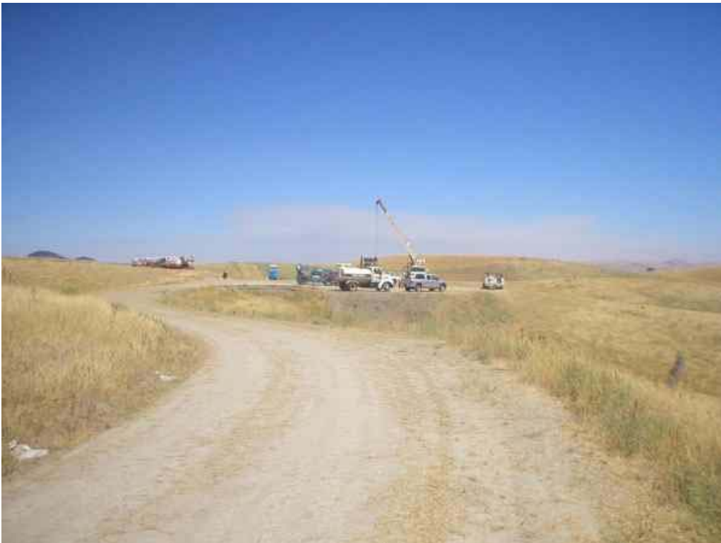
Figure 2 – Cable pulling at Vault 6, July 11, 2006.
