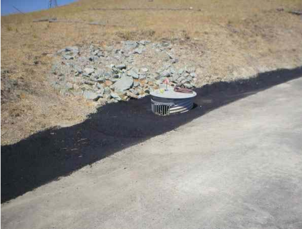
Figure 3 – NVC crews paved v-ditches along Road 6, August 29, 2006.
