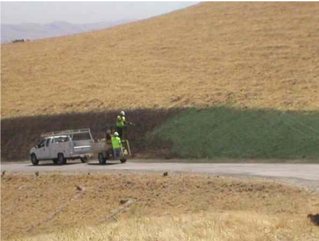
Figure 2 – With restoration work completed, NVC crews hydro-seeded upslope of Road 6, August 29, 2006.
