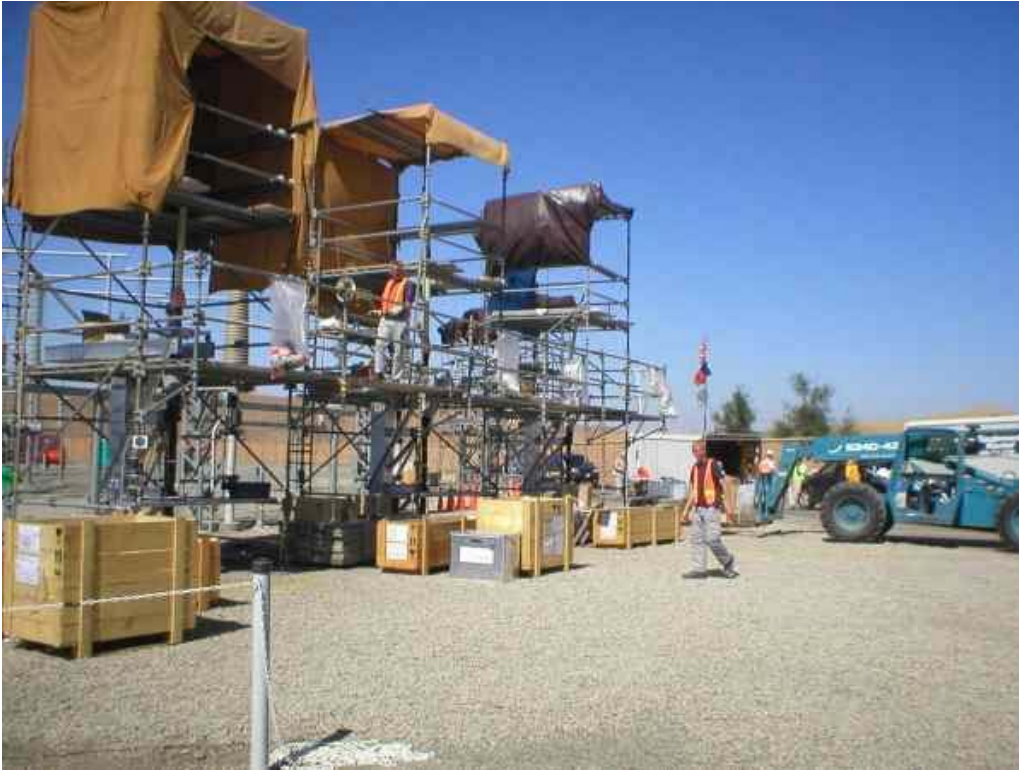
Figure 1 – Crews work on the termination structures at the Cayetano Substation, August 29, 2006.
