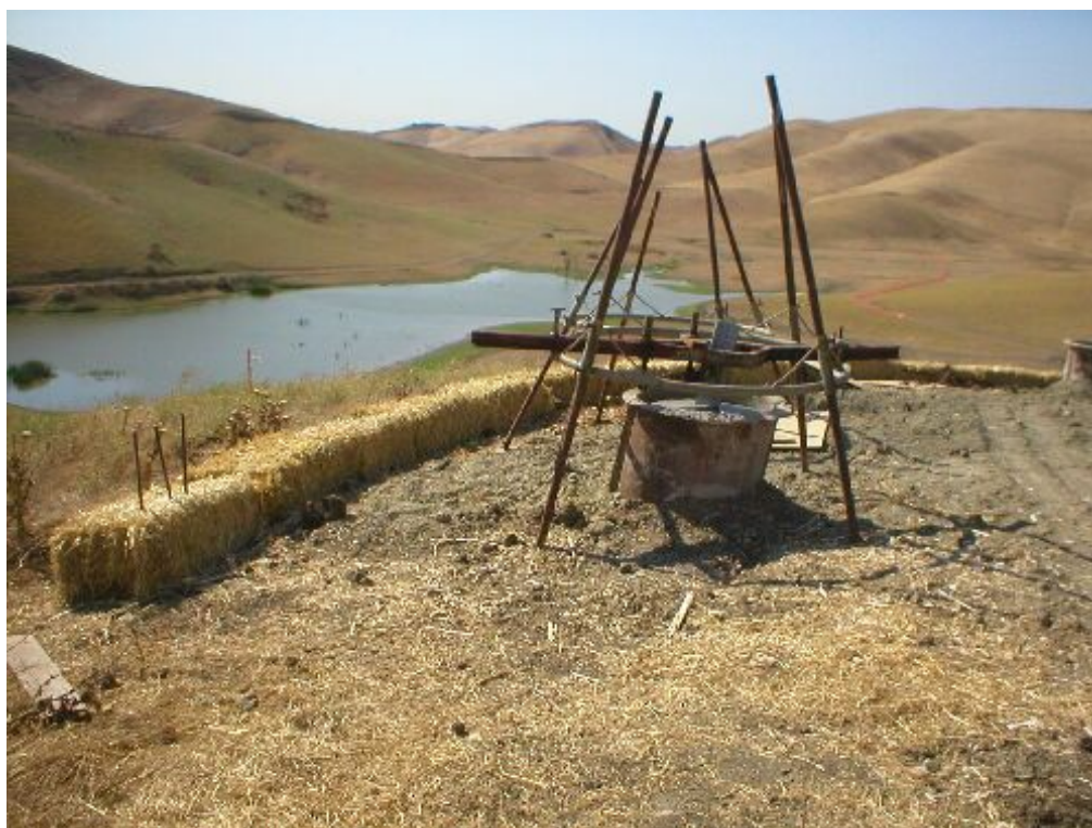
Figure 3 – Foundation construction at Tower #38, Phase Three, July 20, 2005.
