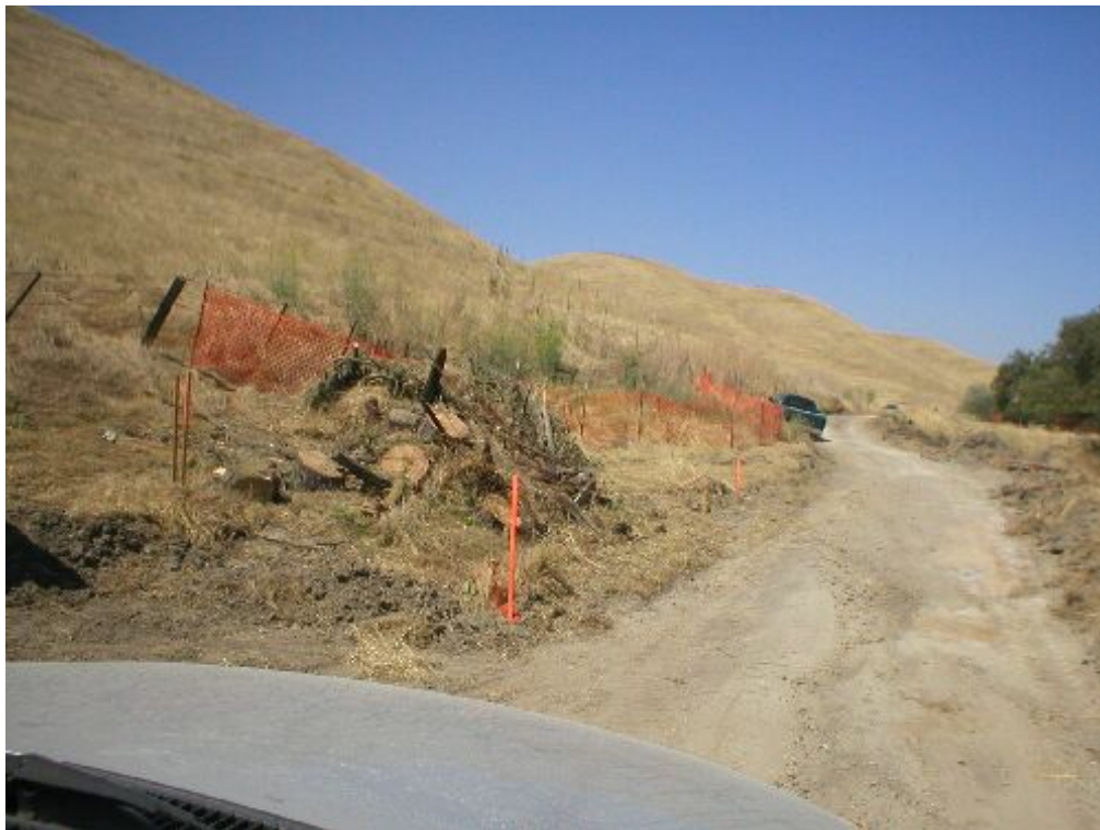
Figure 2 – Tree removal remains along the Moller Ranch Road, Phase Three, July 20, 2005.
