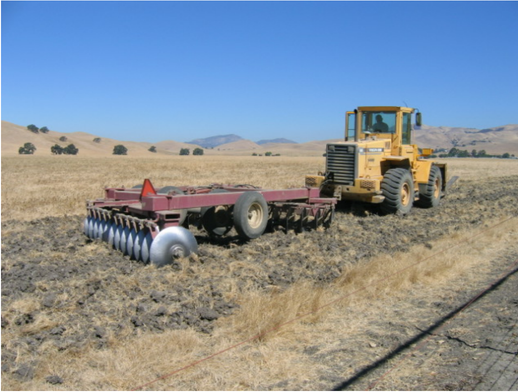
Figure 1 – Construction of the underground portion began August 10, 2005.
