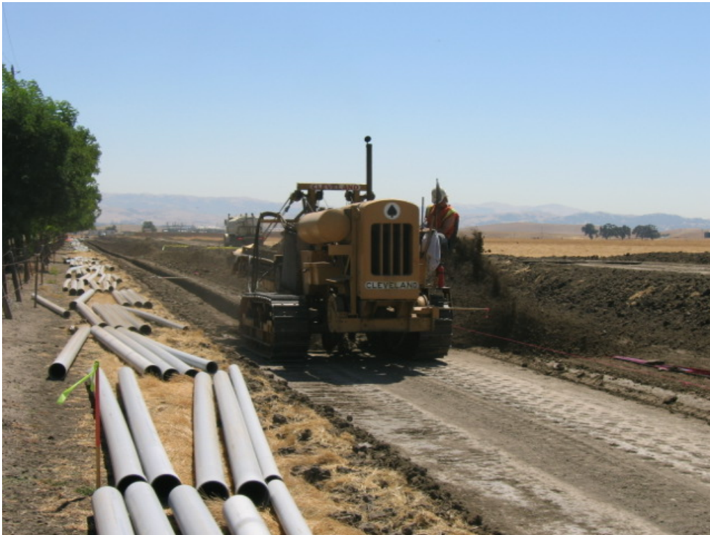
Figure 2 – Trenching continues along North Livermore Ave., August 17 th , 2005.
