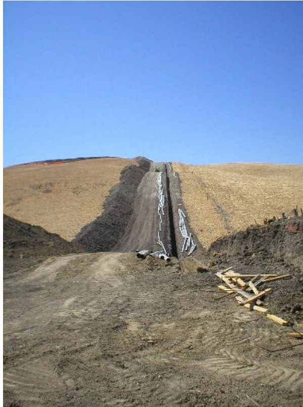
Figure 1 – Trench line proceeding past Road 5 approaching the Transition Station, September 14, 2005.
