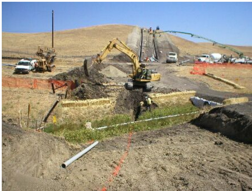
Figure 2 – Trenching operations proceeding through Cayetano Creek, September 14, 2005.
