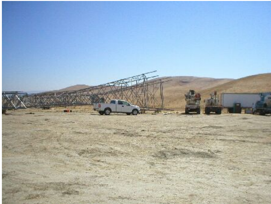
Figure 4 – Tower construction at the Doolan Canyon Laydown area, September 14, 2005.
