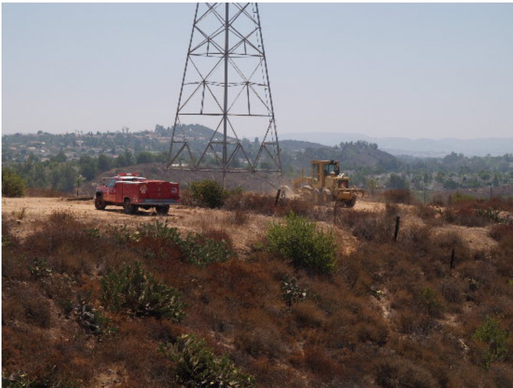
Figure 4 – CDF grader working SCE transmission line easement.
