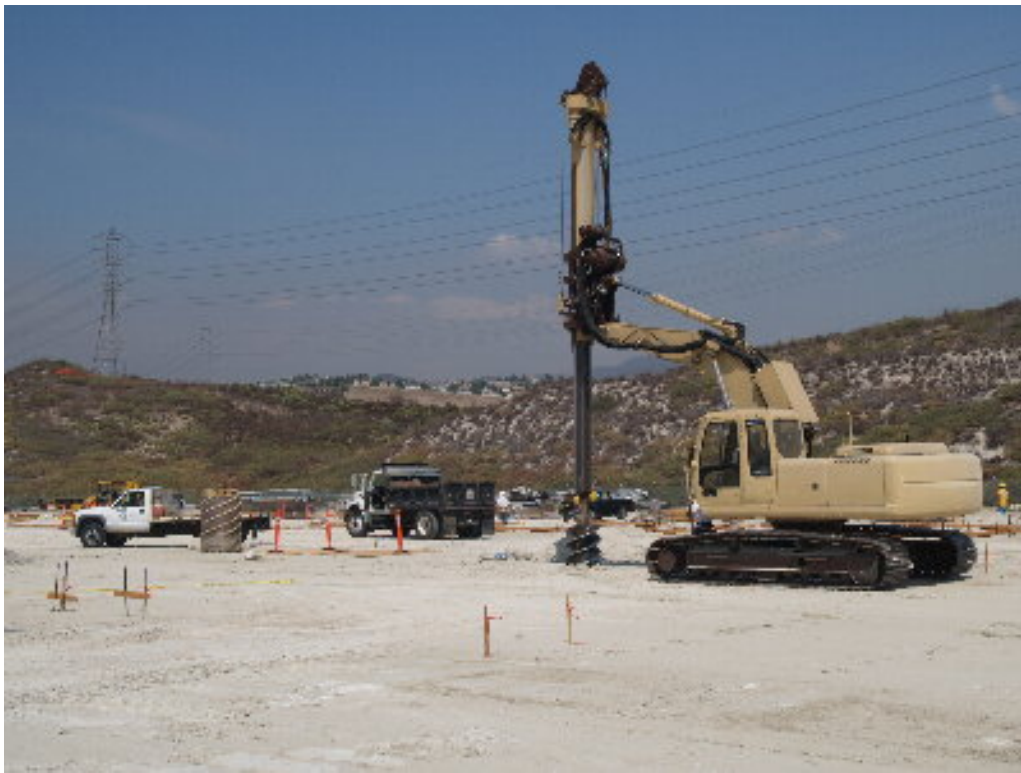
Figure 3 – Drilling continues in the hard material on the substation site.
