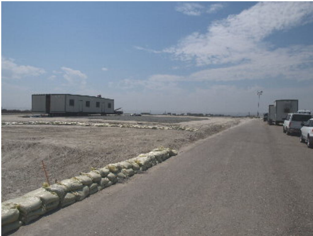
Figure 4 – New office trailers have been delivered to the substation site.
