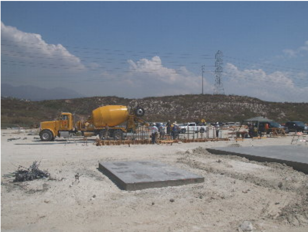
Figure 2 – Several pads have been completed at the substation site.
