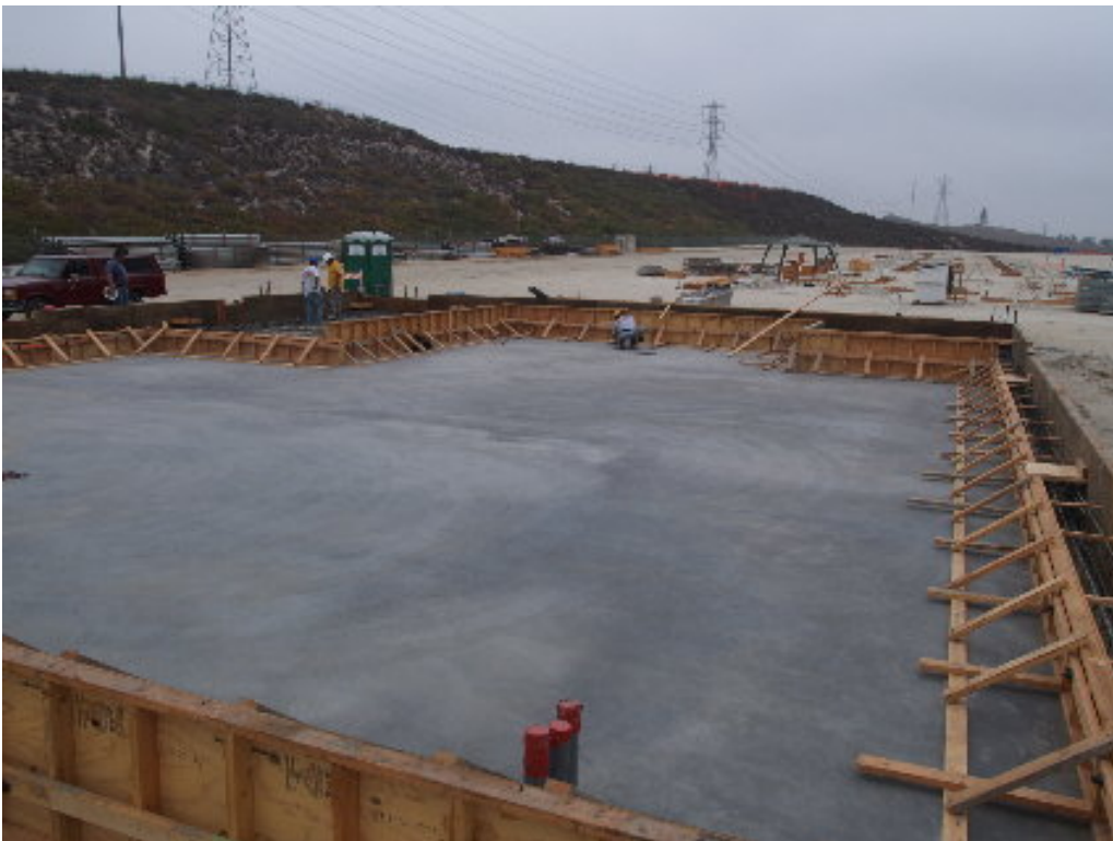
Figure 2 – Completed floor and formwork for the stub walls on the MEER.
