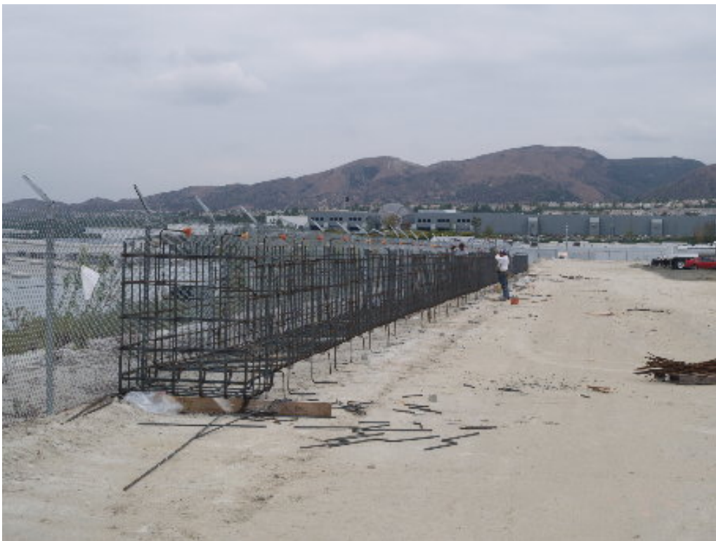
Figure 2 – Ironworkers built the cage for the 300-foot utility trench.
