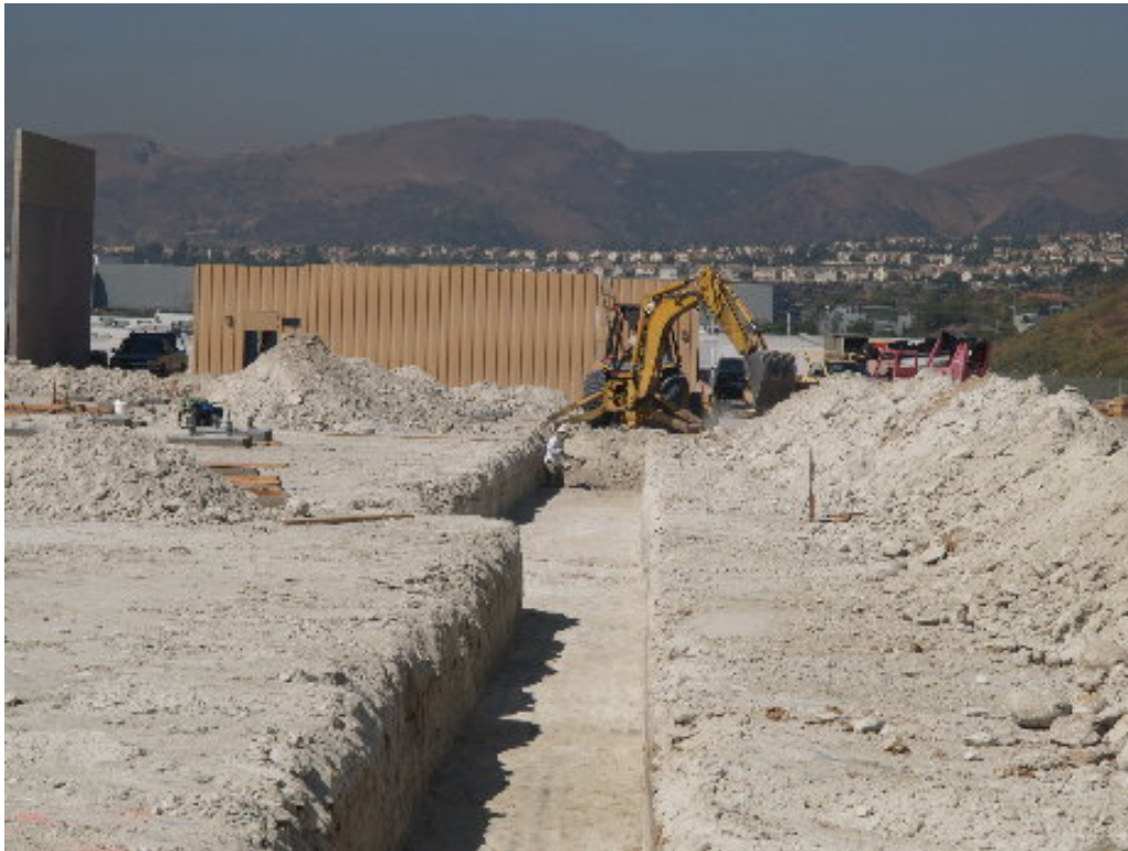
Figure 3 – An operator excavated the main trench leading into the 220 kV MEER #1.
