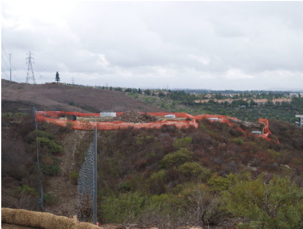
Figure 3 – Several complete foundations on the transmission line right-of-way.
