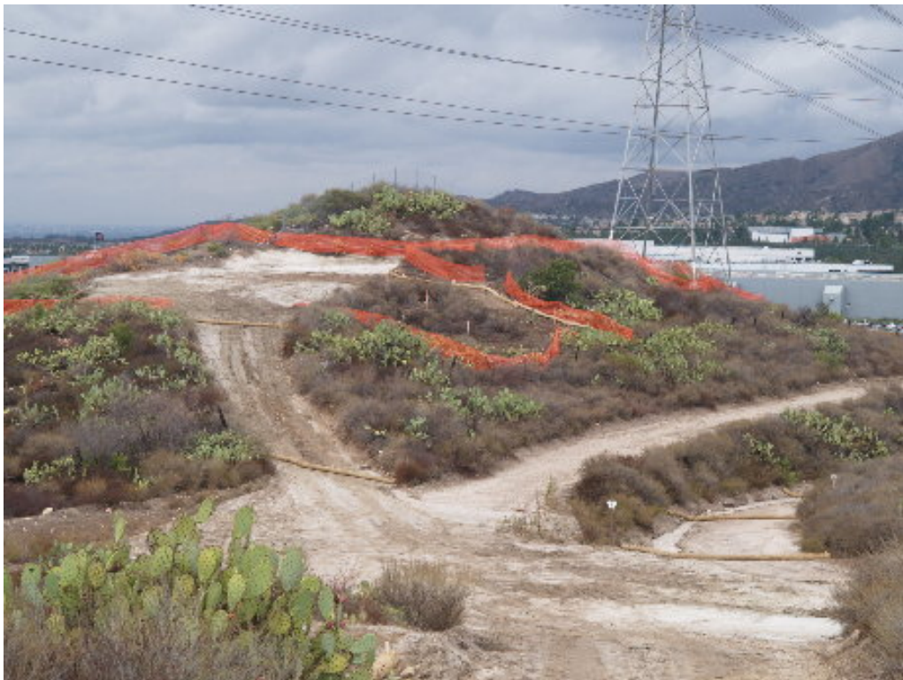
Figure 4 – SCE has installed straw waddles at the pad locations and along access roads on the 220 kV corridor to control erosion and sedimentation.
