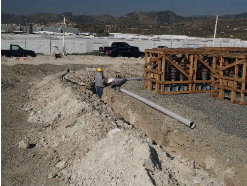
Figure 3 – A crew worked on the fiber-optic conduit within the substation site.
