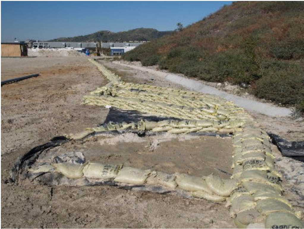
Figure 5 – A series of sediment traps were constructed further to the east after the fence was removed.
