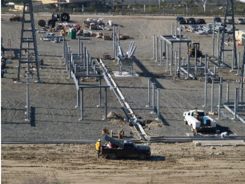
Figure 1 – A small crew worked to connect conduits to the pre-cast trench on the southern end of the substation site.
