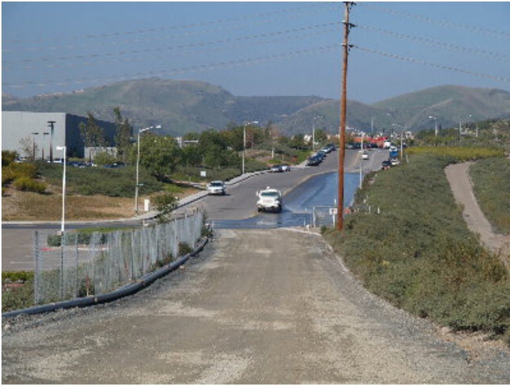
Figure 3 – An operator washed down the road after cleaning off the majority of dust and mud with the sweeper.
