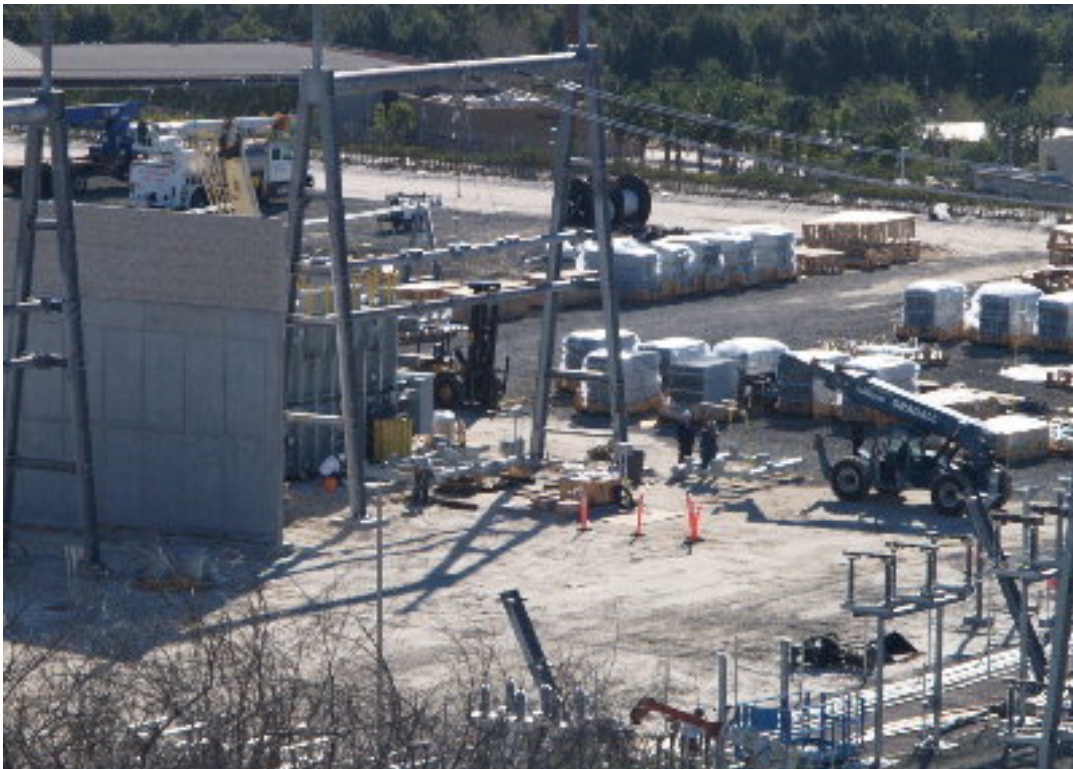
Figure 2 – SCE crews worked to dress the two A-bank transformers.
