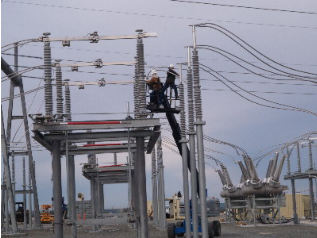
Figure 1 – A small NRG crew worked on the 220 kV bypasses.
