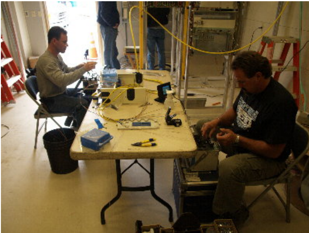
Figure 2 – The fiber optic contractor worked on splicing within MEER #1.
