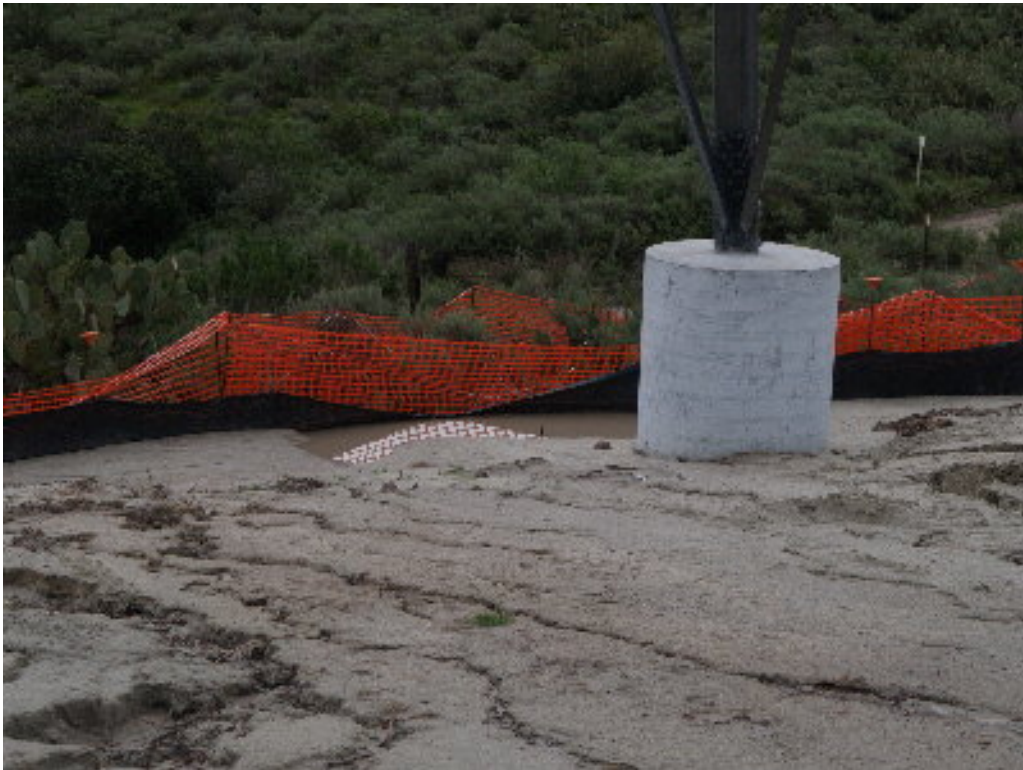
Figure 4 – The silt fencing on the 220 kV transmission line corridor was overwhelmed in several places and requires maintenance.
