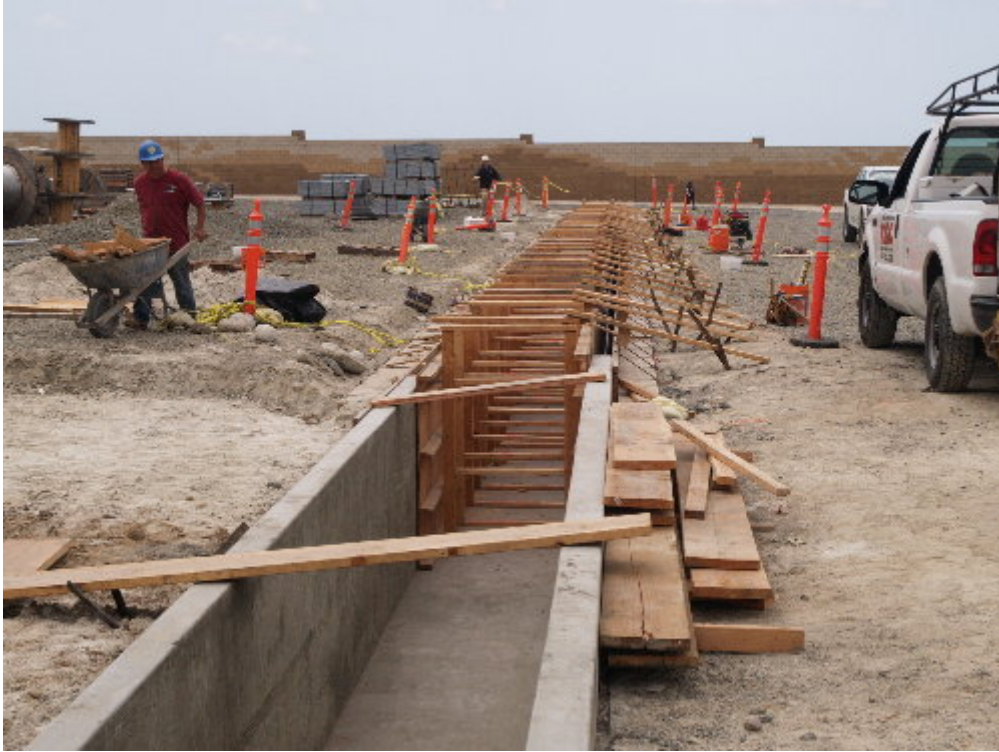
Figure 1 – The second section of the large trench was formed for concrete.
