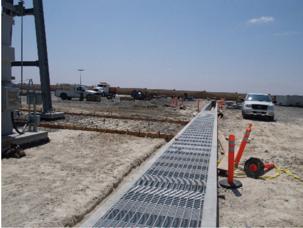
Figure 1 – Crews have installed the steel grate trench covers.
