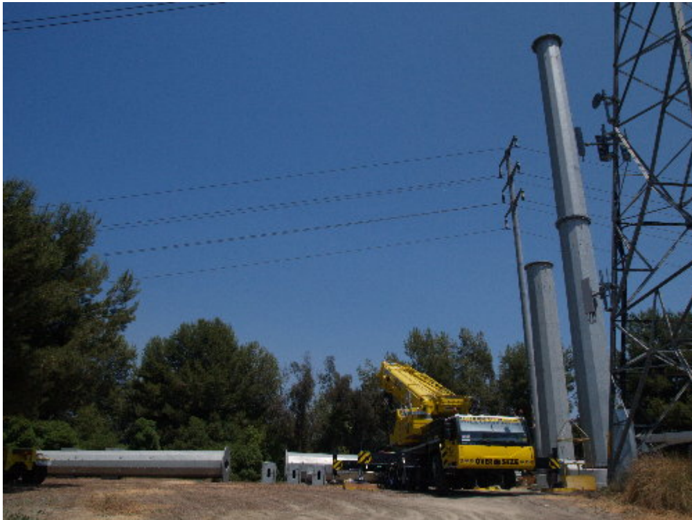
Figure 4 – The Hill Crane was at Structure 7, waiting for work to resume.
