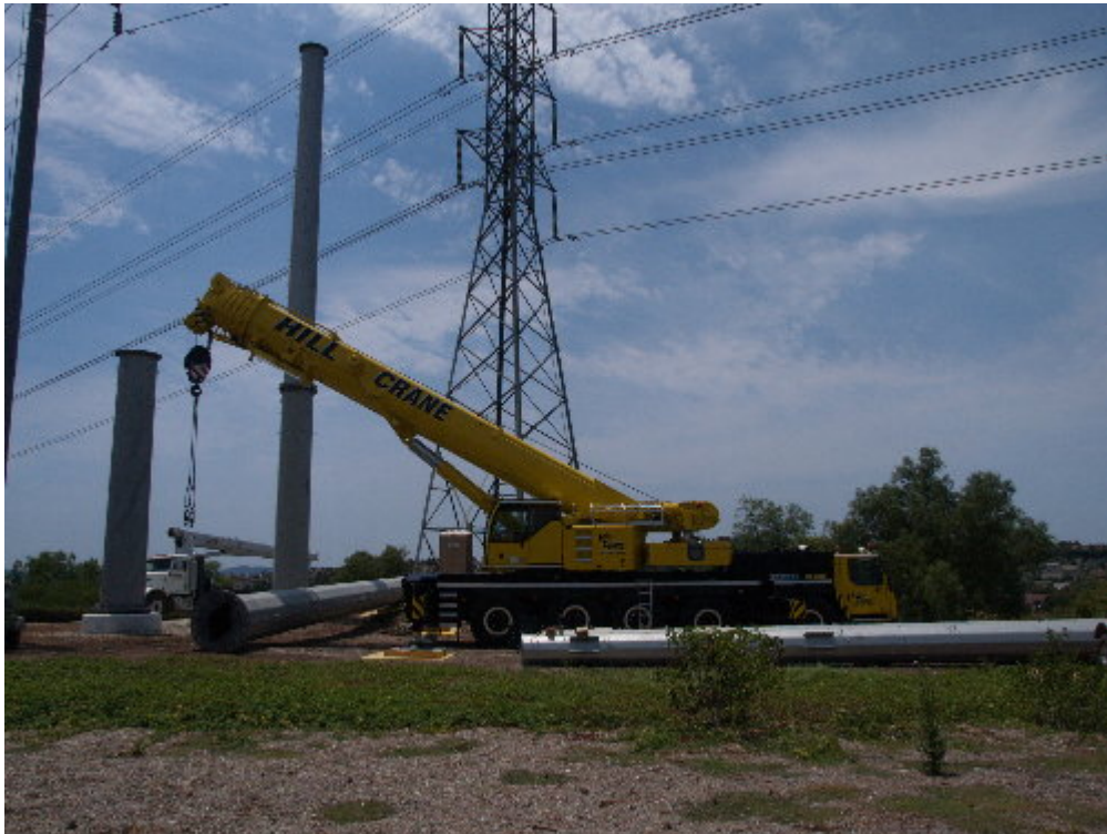
Figure 4 – The Hill Crane was at Structure 6, waiting for work to resume.
