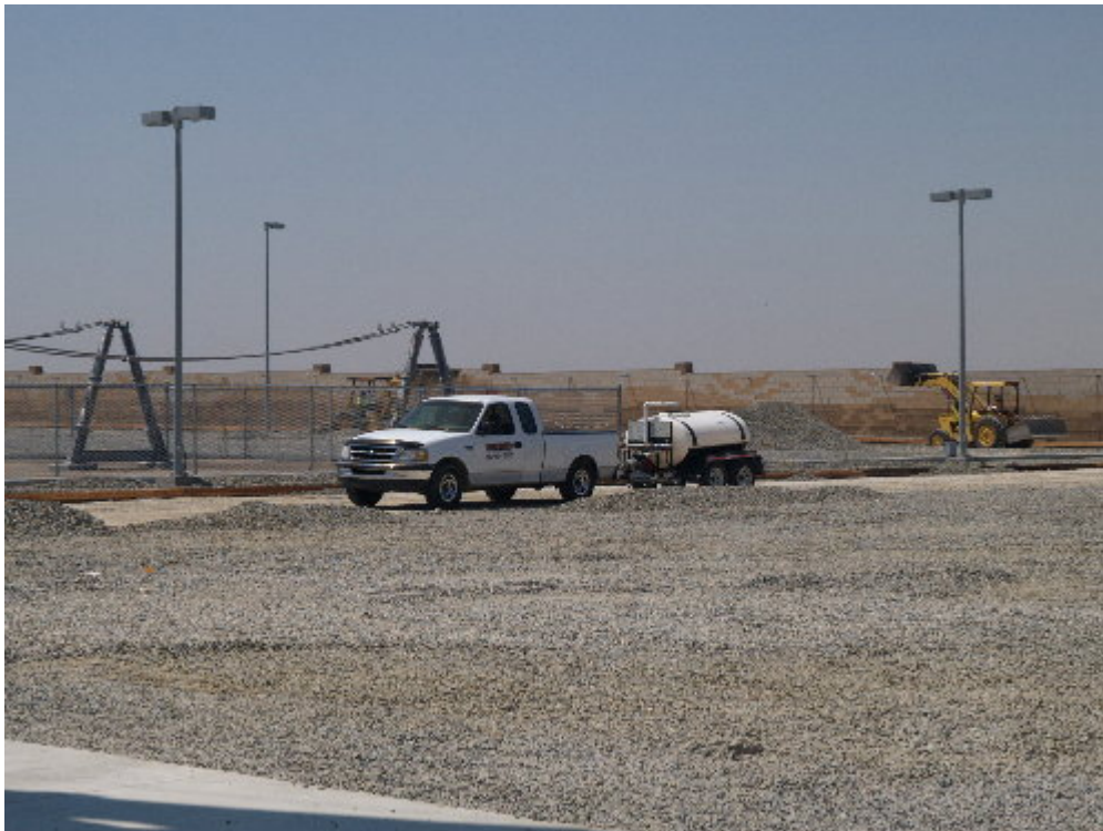
Figure 2 – A small water trailer was used to control dust rather than a water truck during the site visit.
