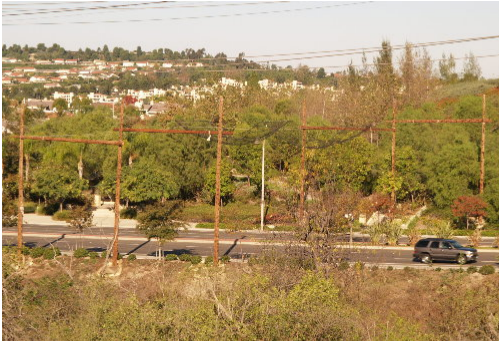
Figure 3 – Netting has been placed between the guard structures at Aliso Parkway to protect the trees in the median.
