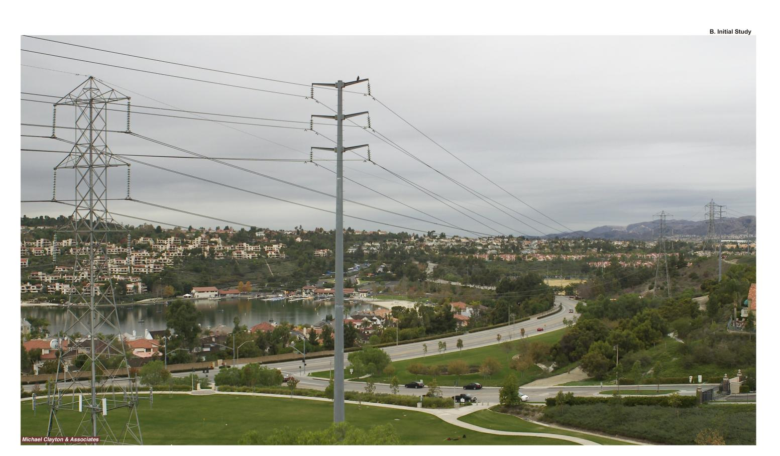
The **existing view** to the northwest from Key Viewpoint 5 at a residence on Sweet Meadow, southeast of the proposed Tower HF-03 location. This view encompasses the existing 66 kV MO-P6 (closest), -P7, and -P8 tower locations. These single-pole 66 kV towers would be replaced with the corresponding double-pole H-Frame 66 kV towers HF-03, -04, and -05.
