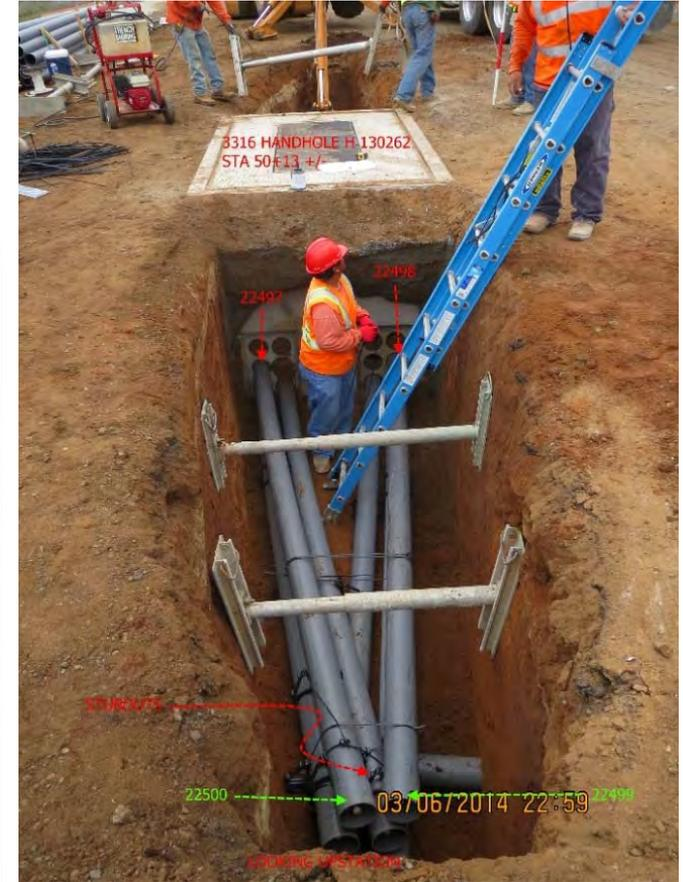
B. Typical 12-kV Duct Bank
