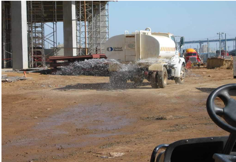
Water being applied for dust control.
