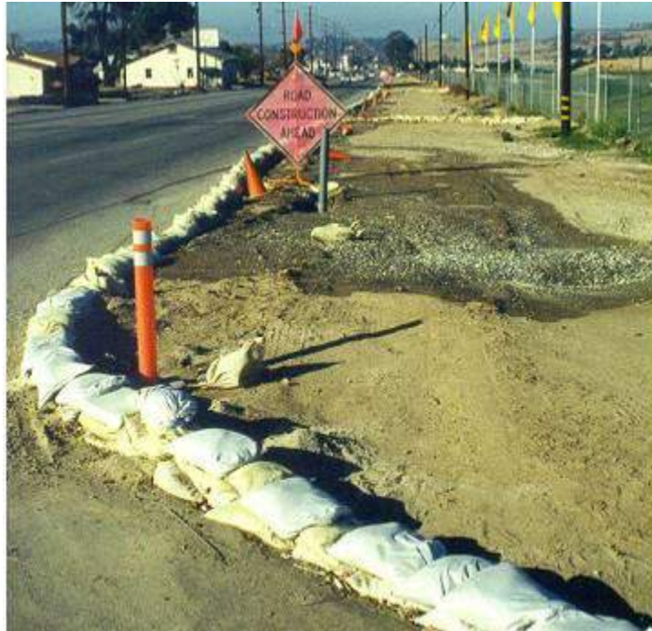
Sand bags used as perimeter control.
