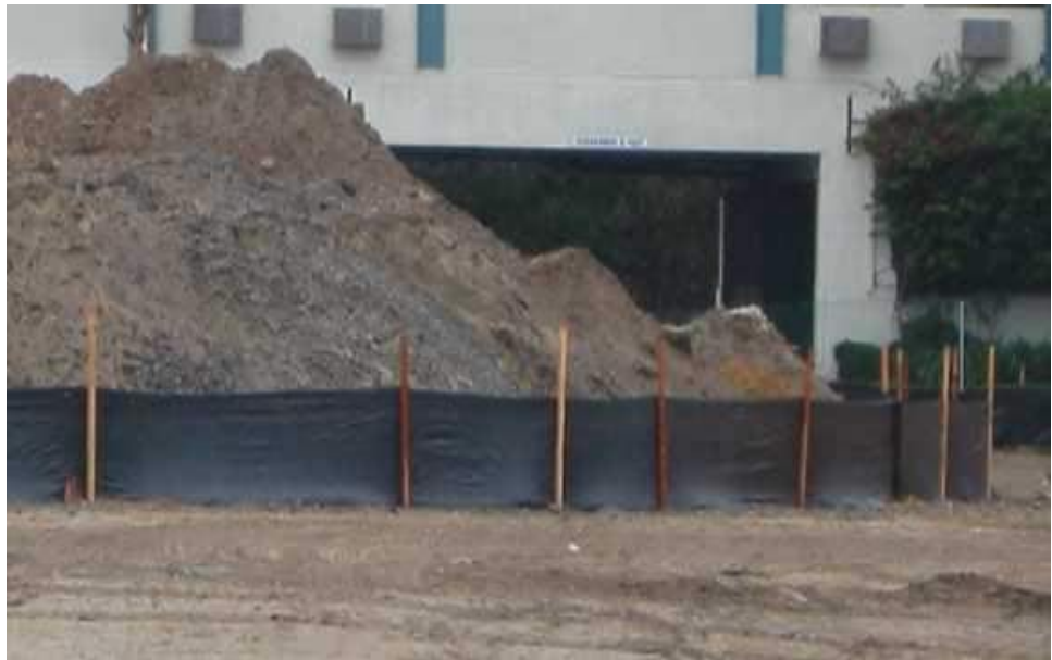
Silt fence used for stockpile perimeter control.
