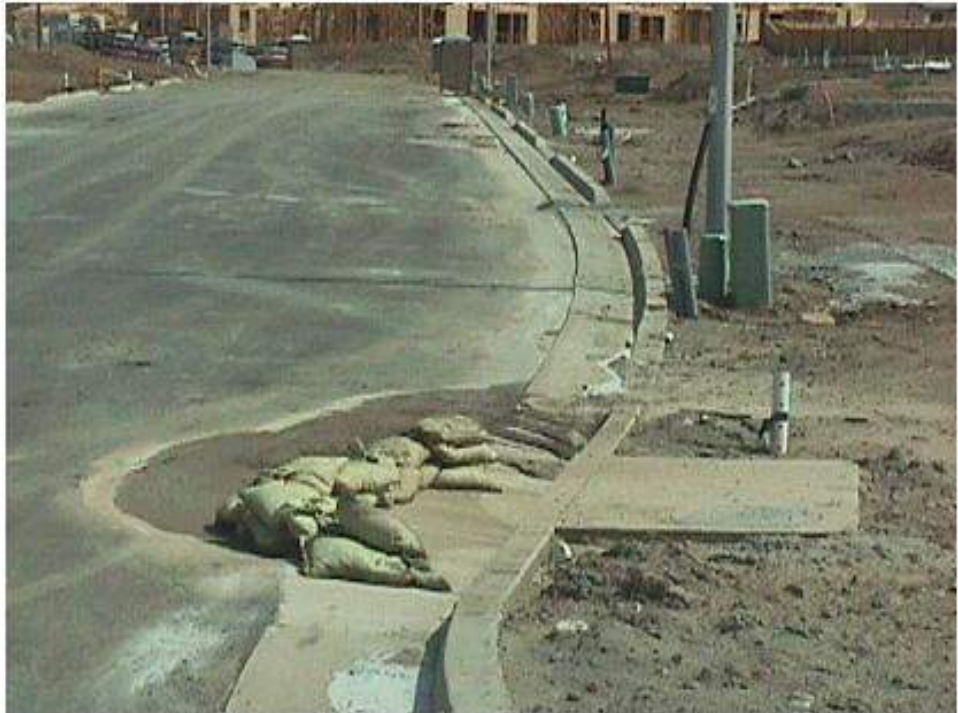
Gravel bag inlet protection.
