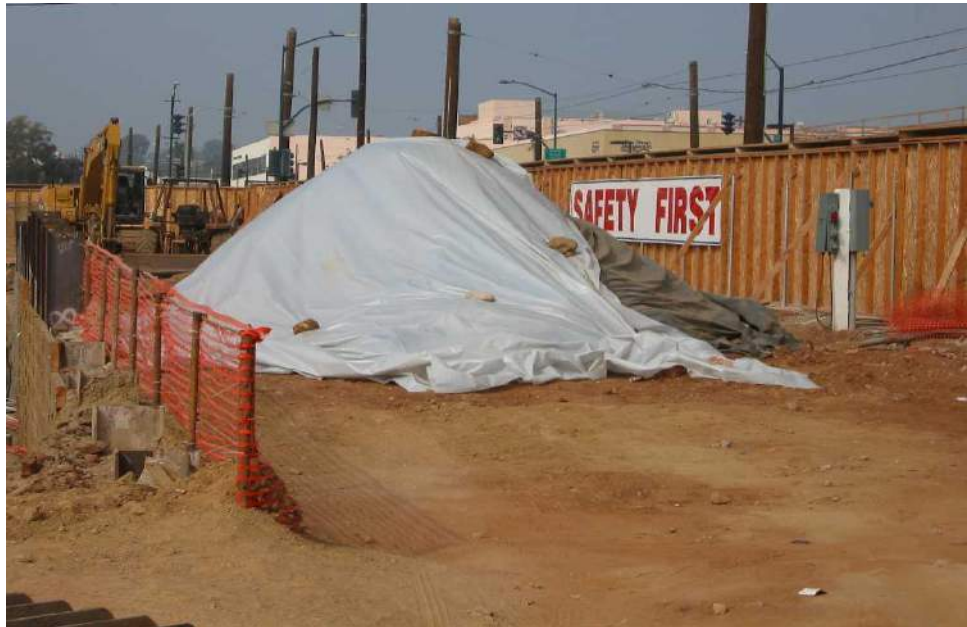
Stockpile covered with plastic and secured with large rocks.
