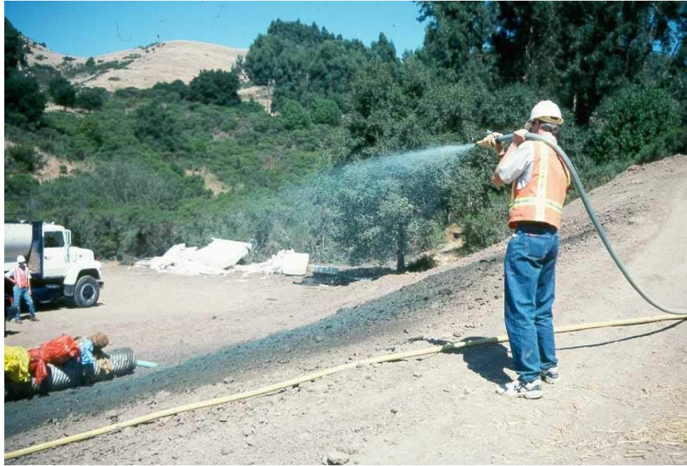
Applying hydroseed.
