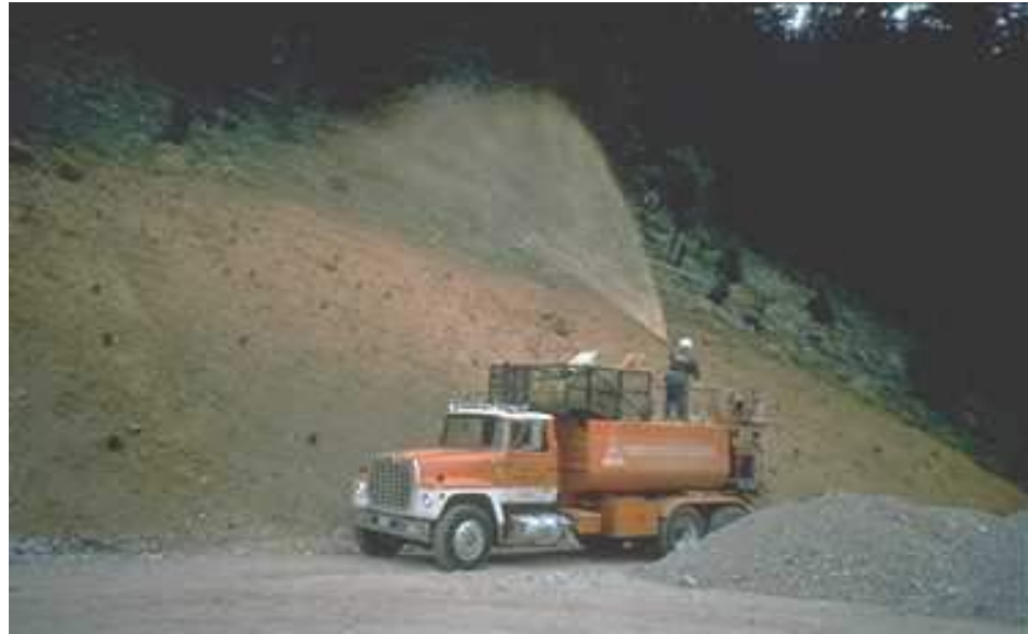
Applying hydraulic mulch.
