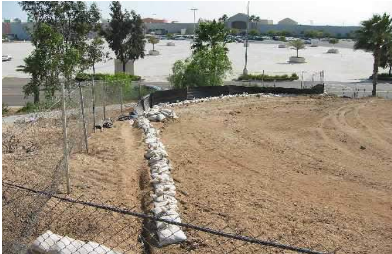
Gravel bags used as perimeter control.
