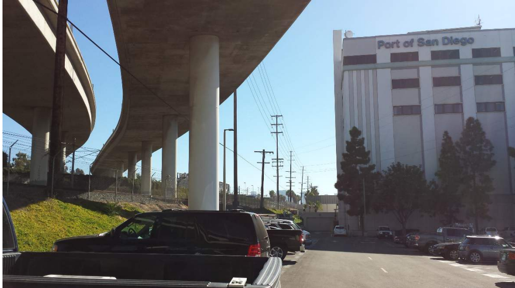
Photograph 5: View of the Port of San Diego building facing south. The Port of San Diego building is located approximately 350 feet west of the 12 kV distribution relocation and approximately 1,100 feet south of the proposed Vine Substation.
