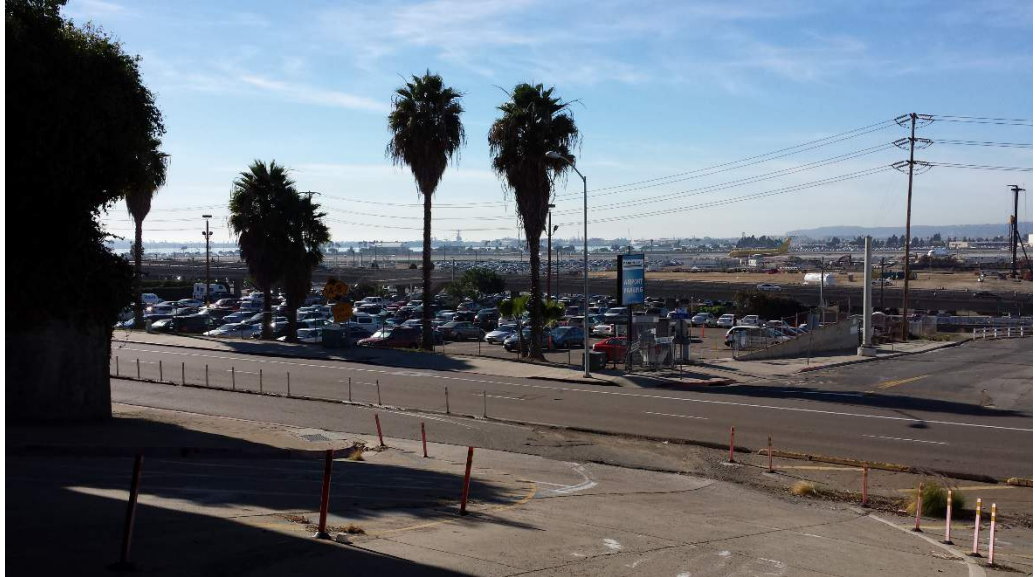
Photograph 1: View of the proposed Vine Substation site facing southwest from Vine Street.
