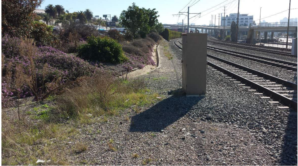
Photograph 3: Ornamental vegetation and a concrete channel located between the proposed Vine Substation site and railroad tracks looking south.
