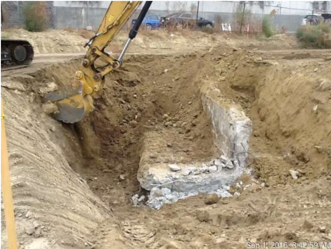
Figure 1 – Demolition of the concrete foundation identified at the Vine Substation site.
