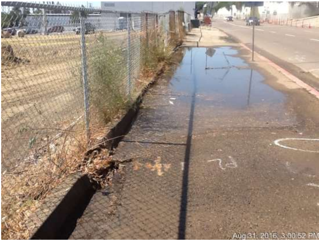
Figure 4 – Water from an accidental release of hydrant water pooled up along Kettner Boulevard.
