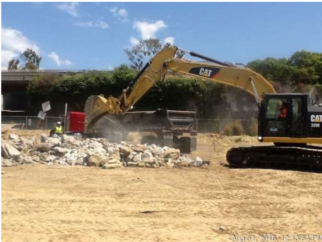
Figure 2 – The foundation was crushed into pieces and hauled offsite for disposal.
