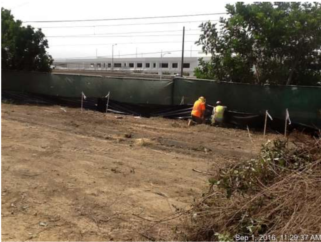
Figure 3 – Temporary fence installation along the railroad right-of-way.
