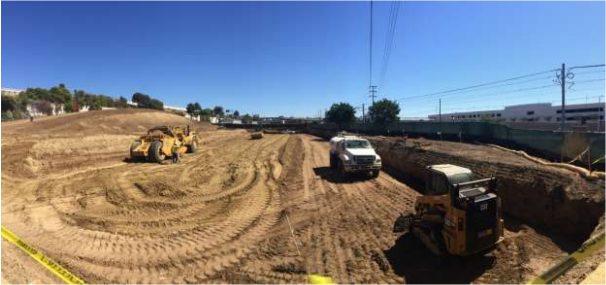
Figure 1 – Mass grading operations in process at the Vine Substation site.
