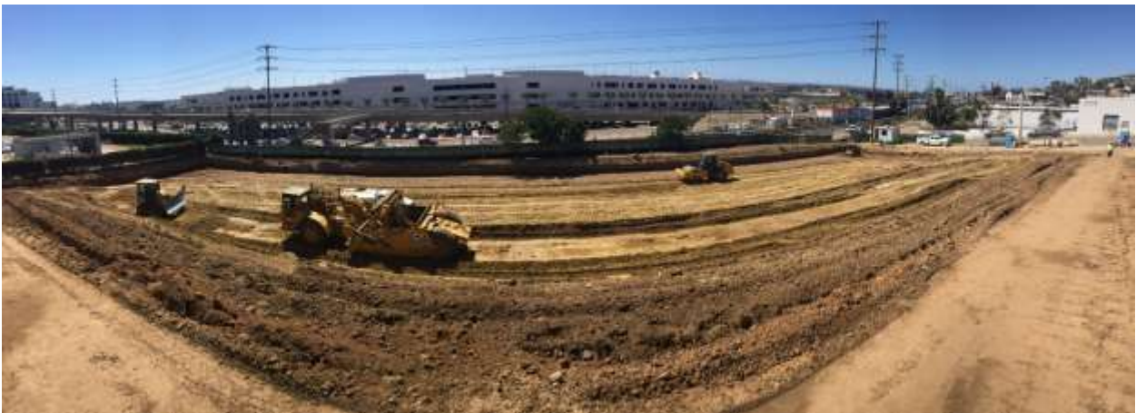
Figure 2 – Mass grading operations in process at the Vine Substation site.
