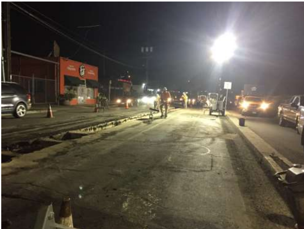
Figure 2 – NPL crews working within traffic control areas along India Street.
