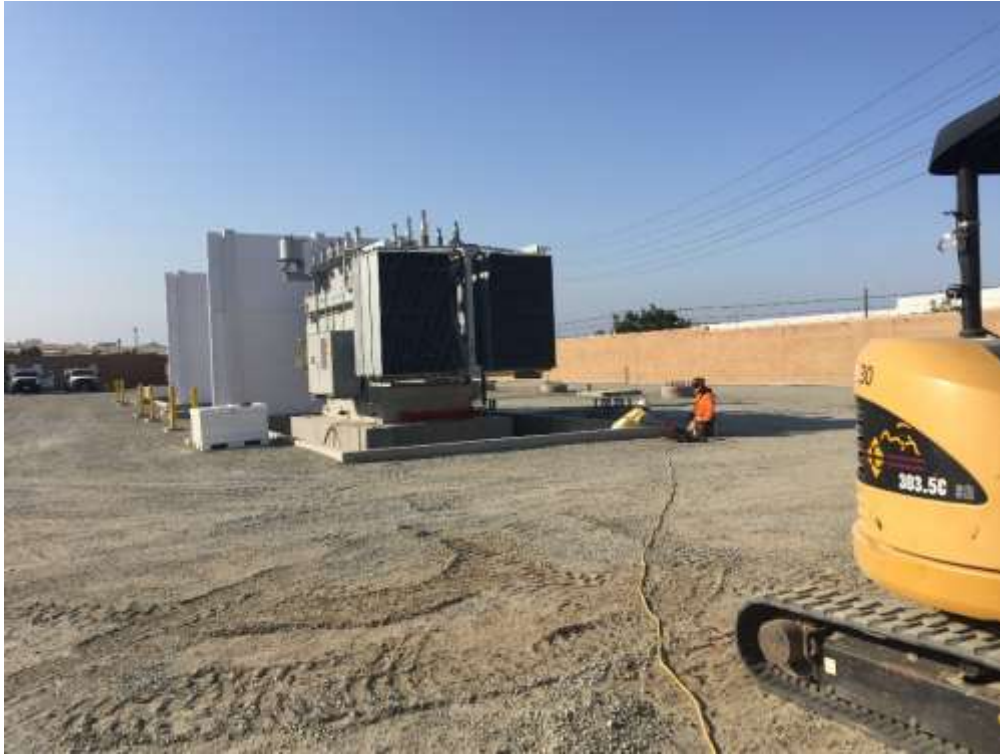
Figure 1 – Kearney crews continued with component installation at the Vine Substation.
