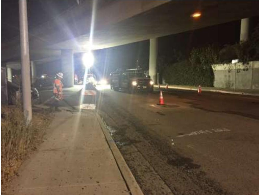
Figure 1 – NPL crews used leaf blowers to remove dislodged cold mix from the sidewalks adjacent to Kettner Blvd.
