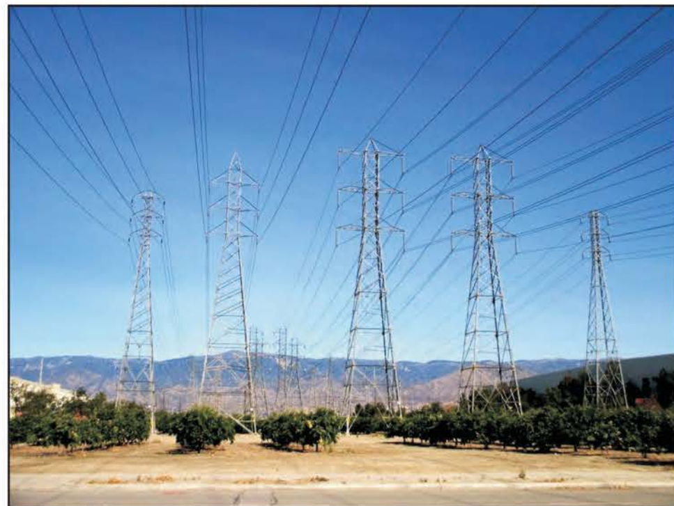
Photo 1. Segment 1 looking south from San Bernardino Substation
