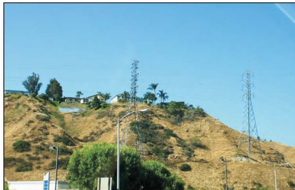
Photo 4. Segment 2 in Colton by Vista Grande Way
