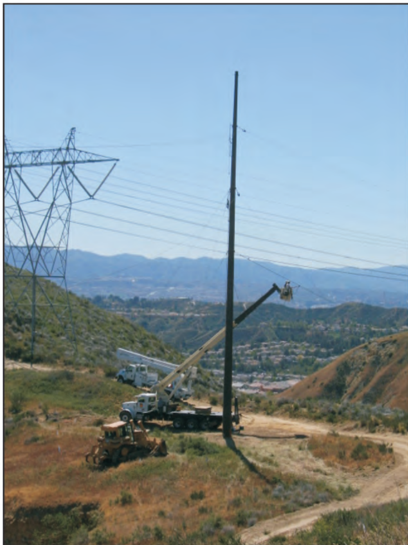
Photo 1. Wire installation on a shoo-fly pole.
