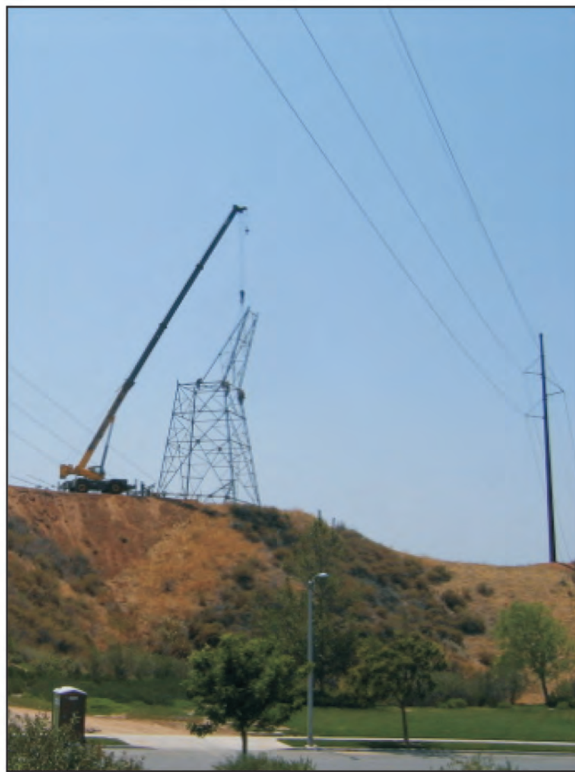
Photo 2. Shoo-fly in use during 220 kV tower removal.
