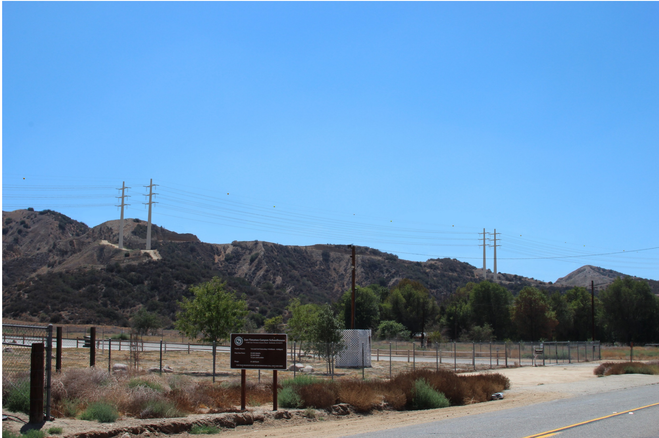
Simulated view that depicts the appearance of a line segment with tubular steel structures constructed using dulled, slightly darkened galvanized steel.
