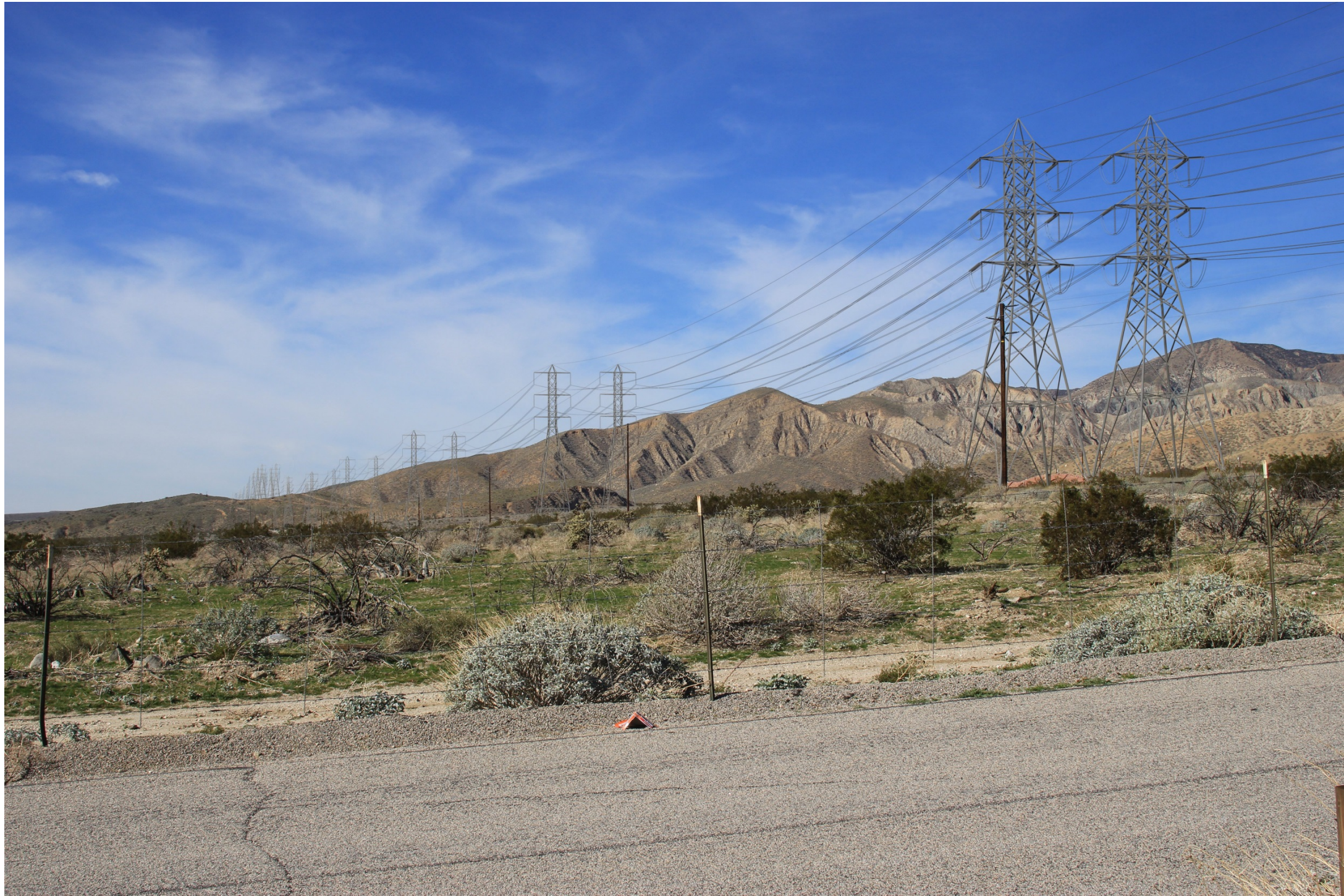
Simulated view that depicts the appearance of a line segment with lattice steel structures constructed using dulled, slightly darkened galvanized steel.
