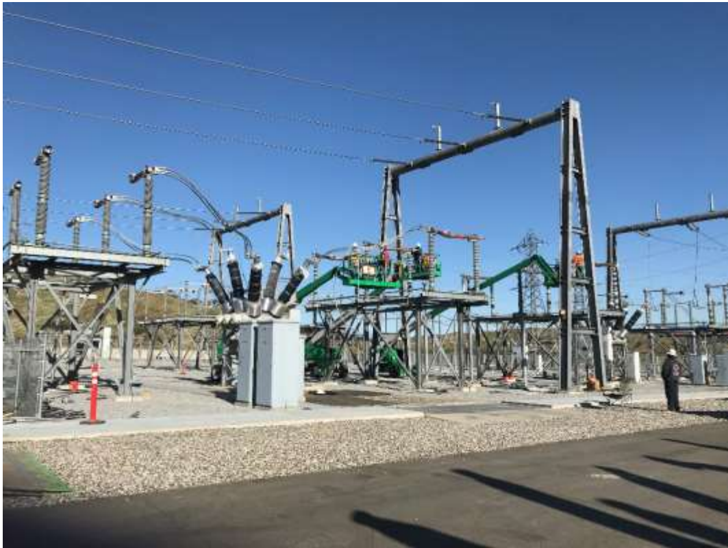
Photo 5 – Crews working at bus position #7 at El Casco Substation (March 27, 2018).
