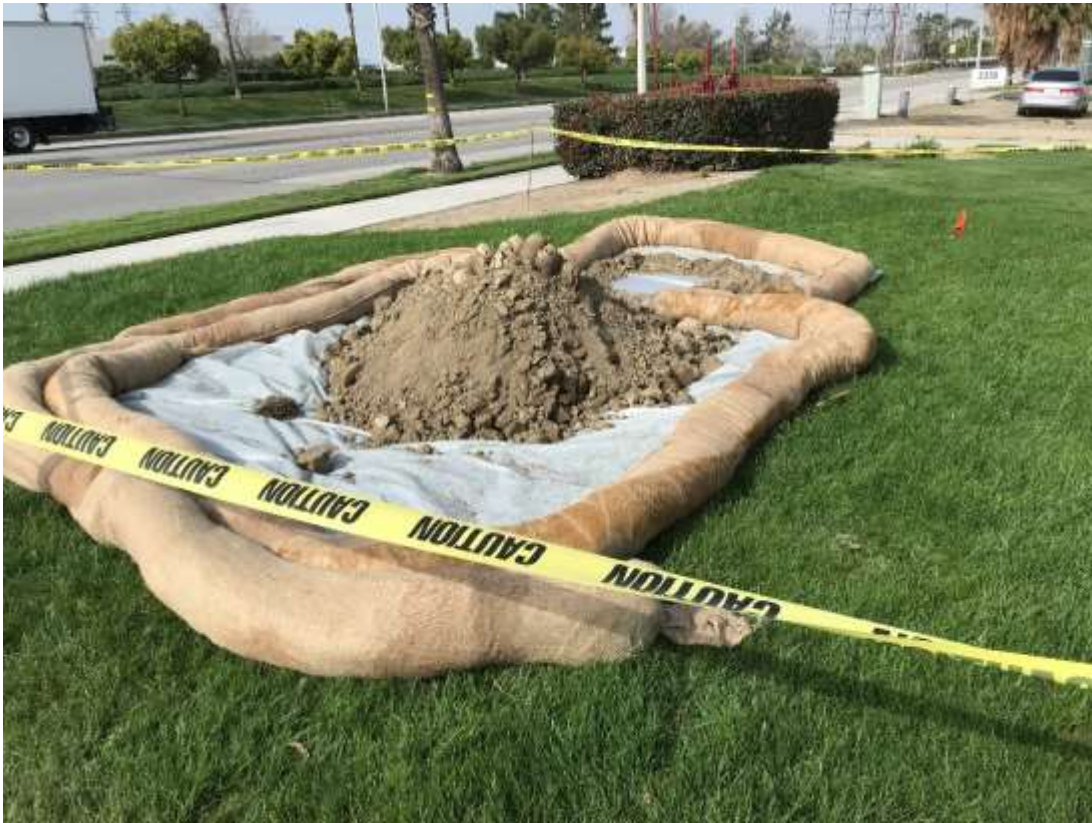
Photo 7 – Lightweight TSP foundation hole properly covered along San Bernardino Avenue (April 6, 2018).
