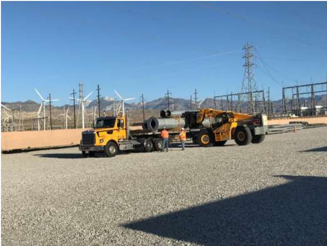
Photo 3 – Materials being transferred from Devers MY to Mountain View MY (March 29, 2018).
