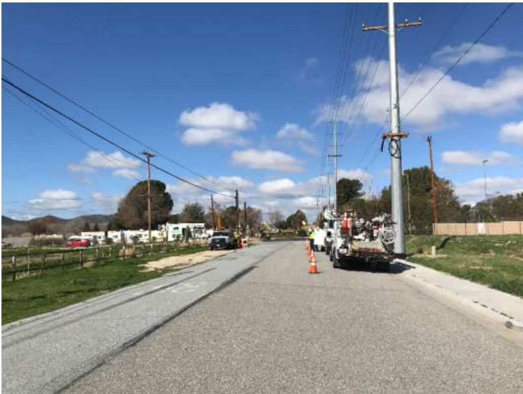
Photo 6 – SCE crew splicing fiber along Wesley Avenue (March 26, 2018).
