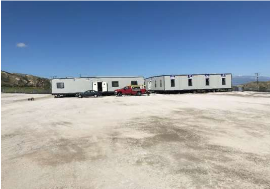
Photo 2 –Installation of office trailers at Poultry MY (March 26, 2018).
