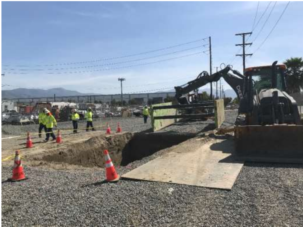
Photo 4 – Excavation complete for vault installation associated with the Timoteo Relocation (April 10, 2018).
