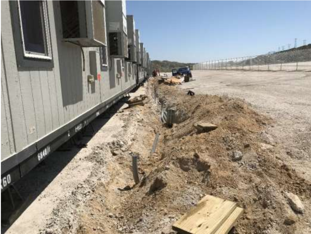
Photo 1 – Installing conduit for telecommunication fiber at the Poultry MY (April 9, 2018).
