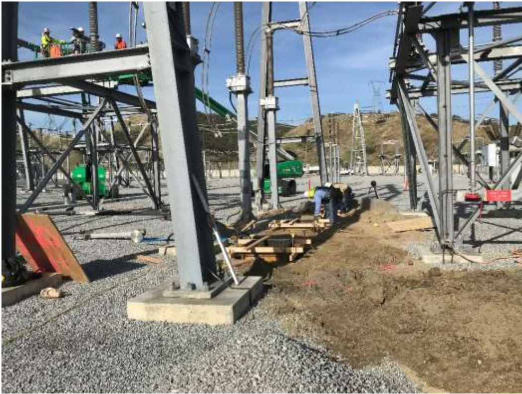
Photo 3 – Framing for new foundations at Position #7 at El Casco Substation (April 10, 2018).
