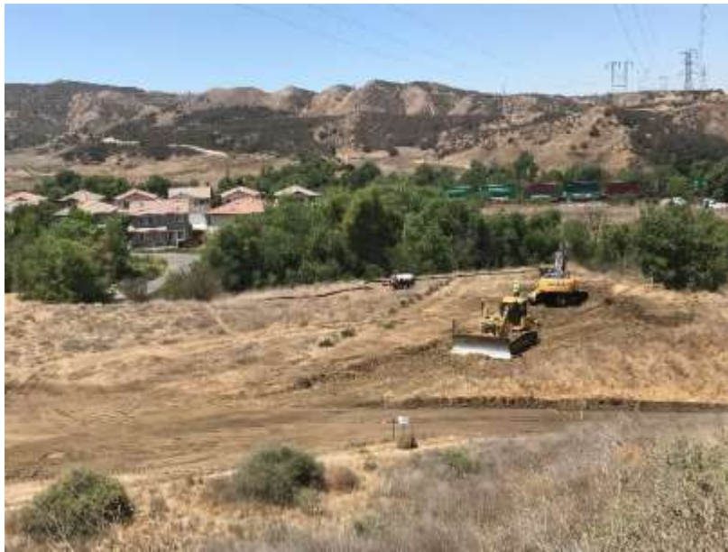
Photo 7 – Grading at Tower Site 4S60 along Segment 4 (June 21, 2018).
