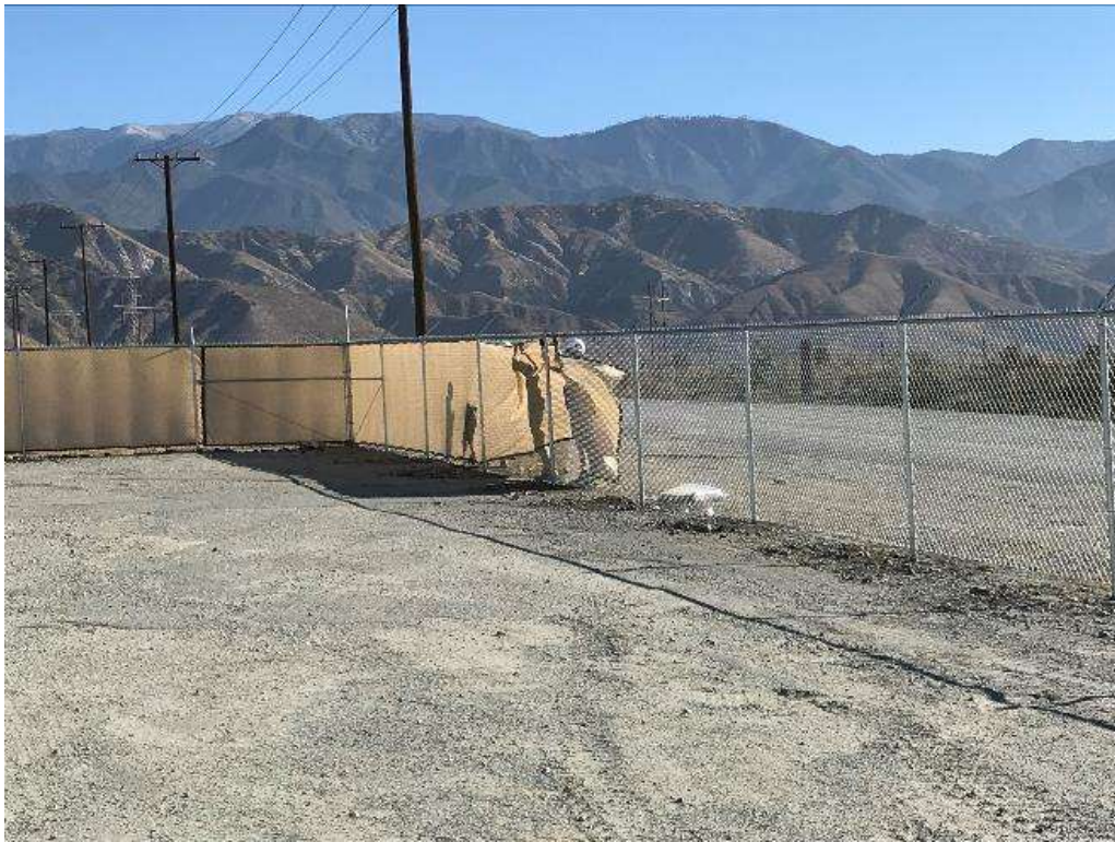
Photo 2 – Installation of privacy screening occurring at Match MY (June 19, 2018).
