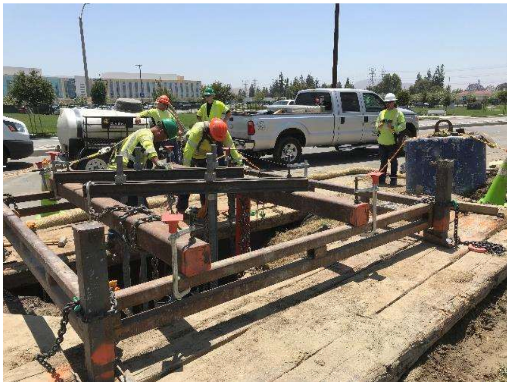
Photo 4 – Foundation excavation at intersection of Redlands Boulevard and Bryn Mawr Avenue for Timoteo Relocation (June 19, 2018).
