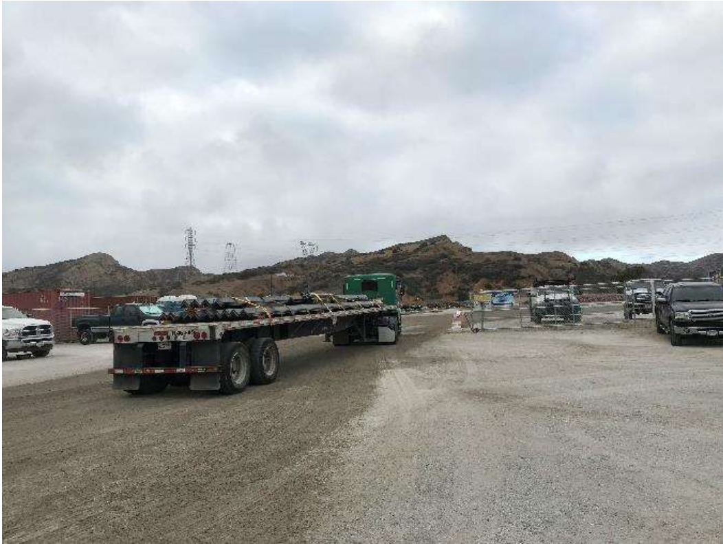
Photo 1 – Delivering stub angle steel to the Poultry MY (June 18, 2018).
