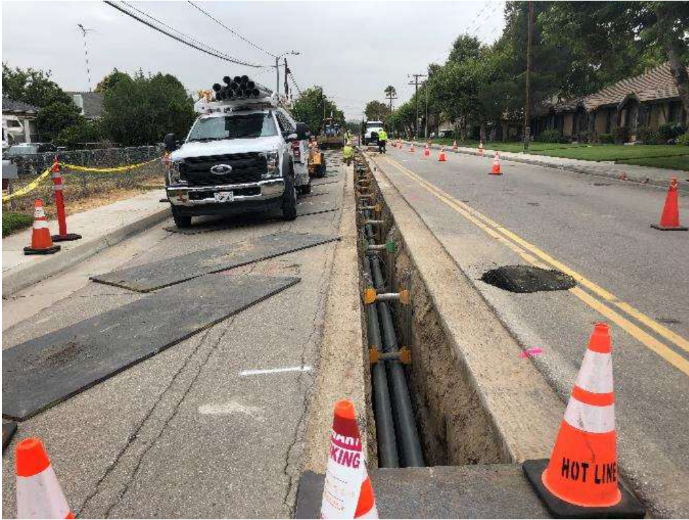
Photo 1 – Installing underground distribution conduit along Mission Road (July 10, 2018).
