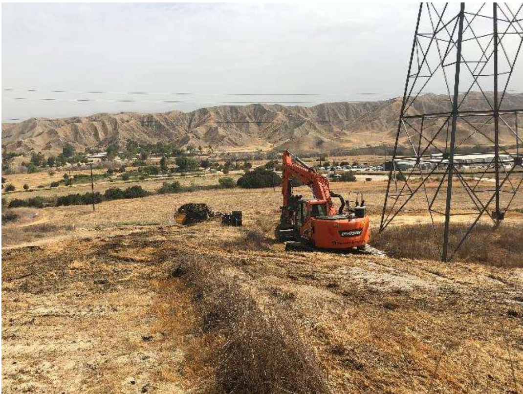
Photo 8 – Grading activities occurring at Tower Site 3X29, transmission Segment 3 (July 10, 2018).
