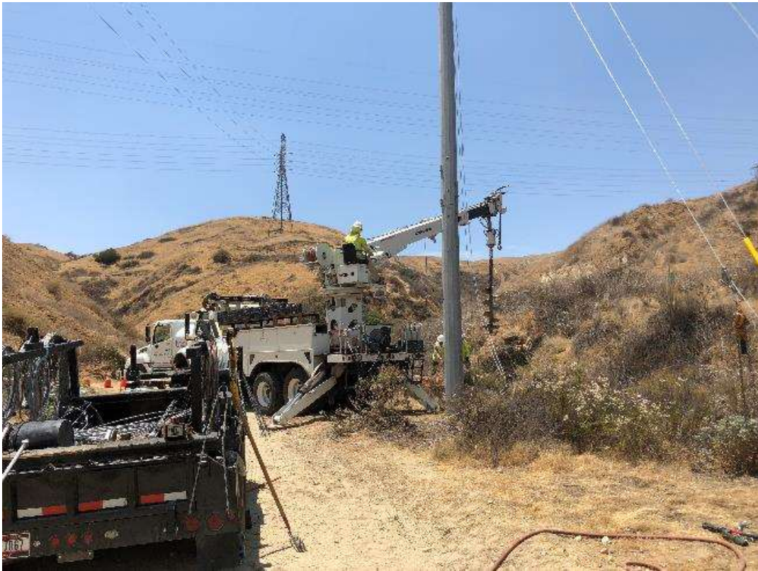
Photo 7 – Installation of one new LWTSP along transmission Segment 2 (July 12, 2018).
