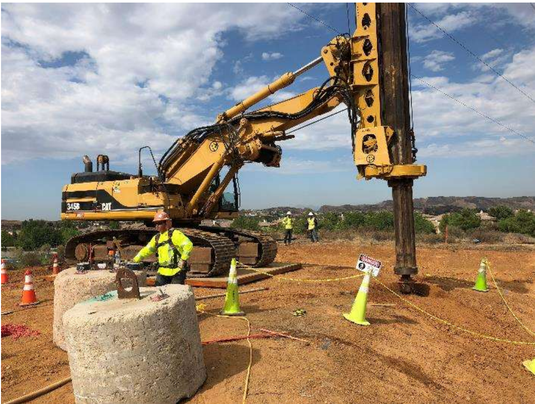
Photo 6 – Foundation drilling at Tower Site 4X48, Segment 4 transmission (July 31, 2018).
