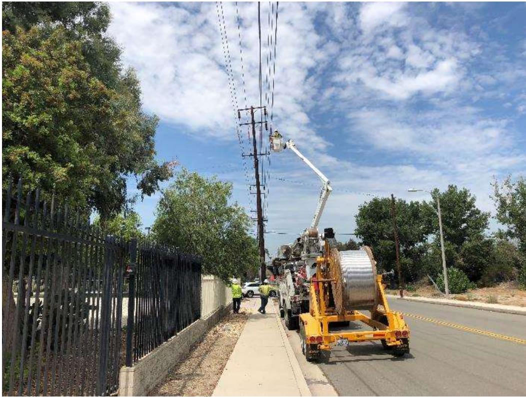
Photo 3 – Replacing conductor along Mayberry Street for Juanita Reconductor (July 30, 2018).
