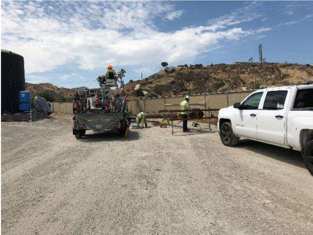
Photo 1 – Installation of wooden distribution pole at Poultry MY (July 31, 2018).
