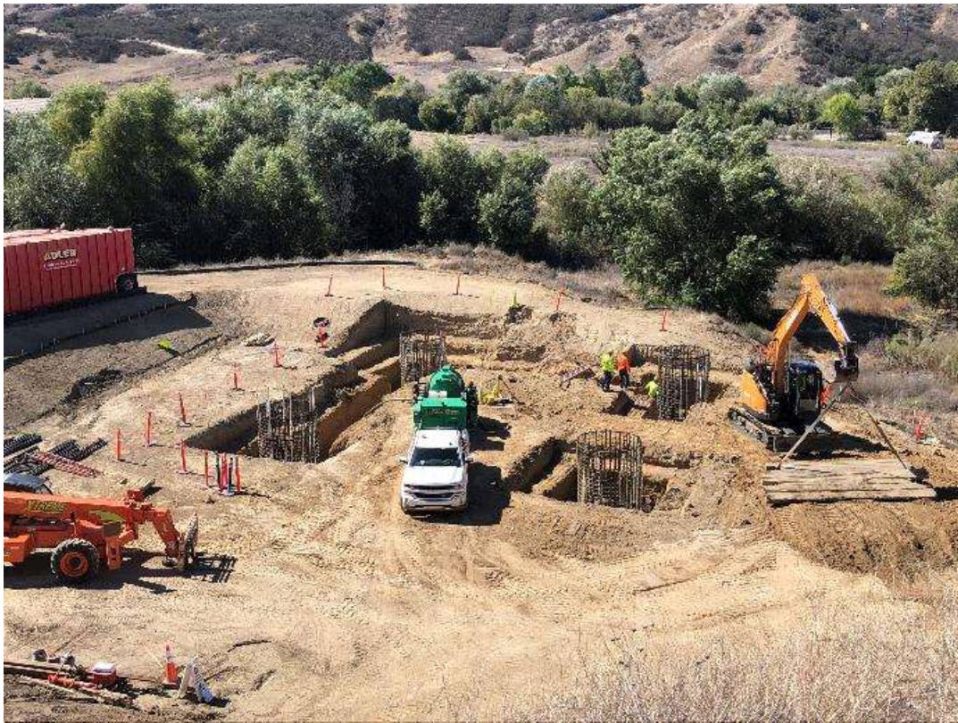
Photo 6 – Grade beam construction at Site 4S60, Segment 4 (October 17, 2018).
