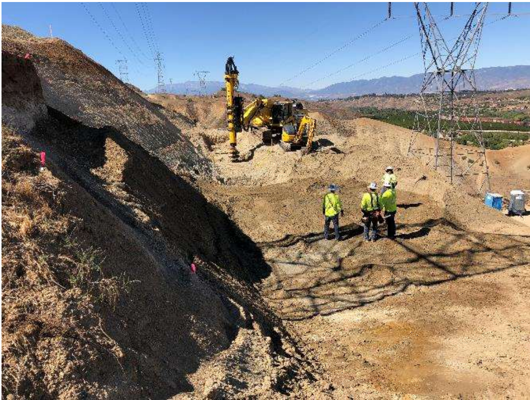
Photo 5 – Foundation drilling for retaining wall at Site 3X37, Segment 3 (October 16, 2018).
