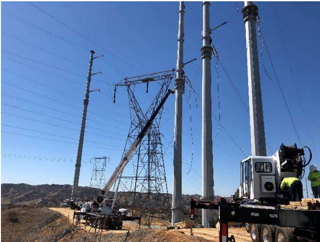
Photo 7 – Transferring conductor wire to shoofly poles at Site 4X56, Segment 4 (October 15, 2018).
