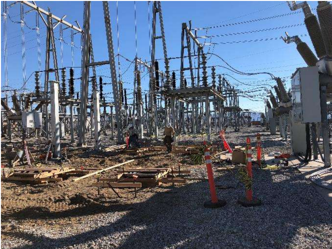
Photo 3 – Forming for new foundations at Position #9 at Devers Substation (October 16, 2018).
