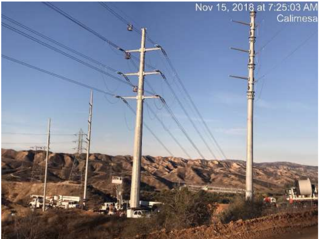
Photo 3 – Wire clipping in Segment 4 (November 15, 2018).
