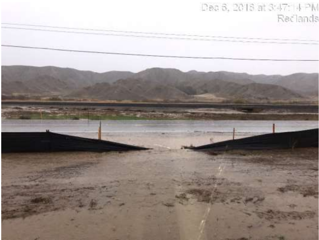
Photo 5 – Storm water breach of silt fencing at the Poultry Yard (December 6, 2018).
