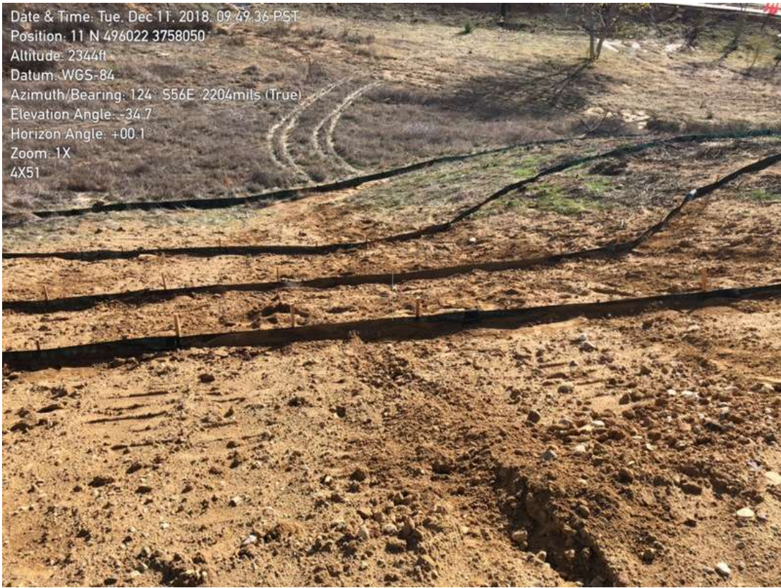
Photo 9 – Conditions after excess sediment clean-up at Site 4X51. Photo courtesy of SCE.
