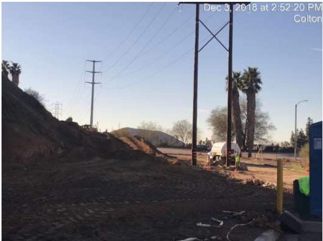
Photo 4 – Access road construction in Segment 2 to Site 2X32. Paleontological monitors are required due to highly sensitive substrate.
