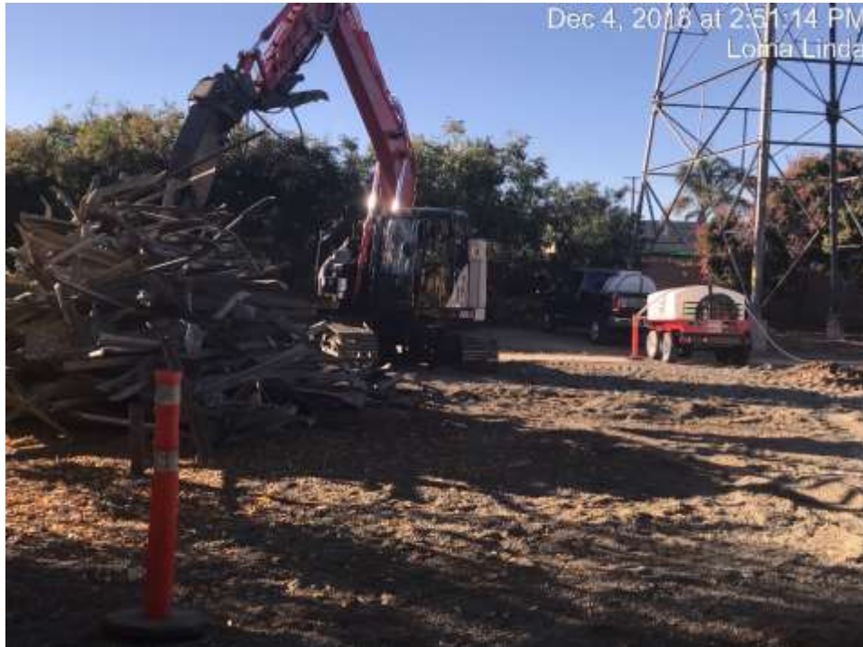
Photo 1 – Tower removal in Segment 1, part of the current outage work (Move 1).
